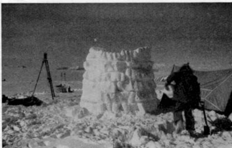
Photo 14. Building a survey cairn of snow blocks.
