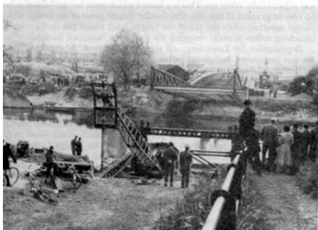
Photo 2. The nose nearing the landing rollers.
