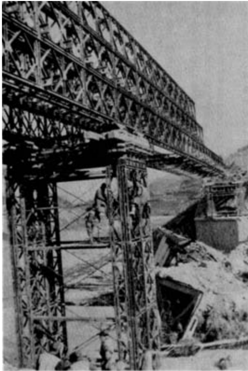
Photo 3. Checking for distortion in the pier and tightening bracing during a pause in launching.
