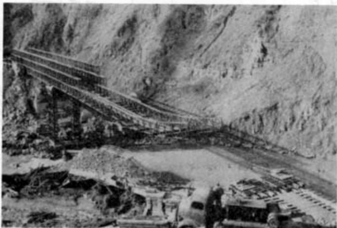
Photo 2. The hauling wire attached. The vehicle in the foreground is a Leroi 250 c fm compressor of which we had three in constant use. In addition to the normal tools it had rip- and crosscut-saws, a pile-driver and a spike hammer.
