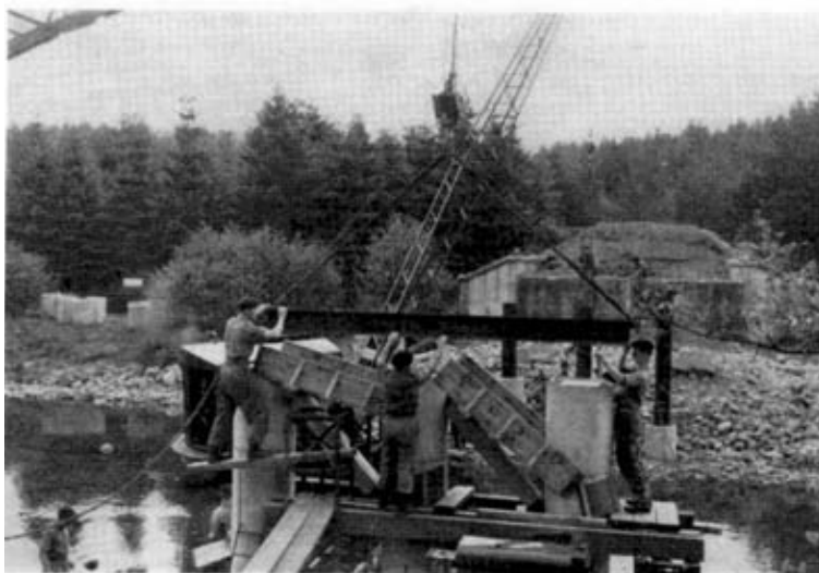
Photo 3. Lowering the capsill on the north pier.
