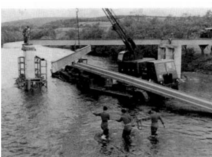
Photo 5. Erecting the main beams.
