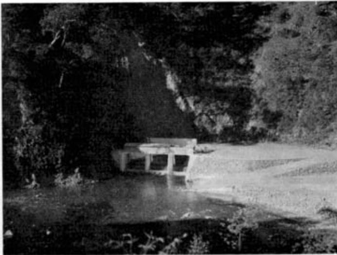
Photo 3. Tailrace Tunnel Outlet Structure with a small discharge to the Tumut River over temporary stoplogs.
