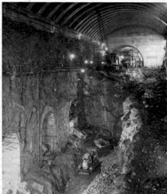
Photo 1. A view towards the Access Tunnel of the Machine Hall during excavation. Penstock portals are on the left of the photograph.
