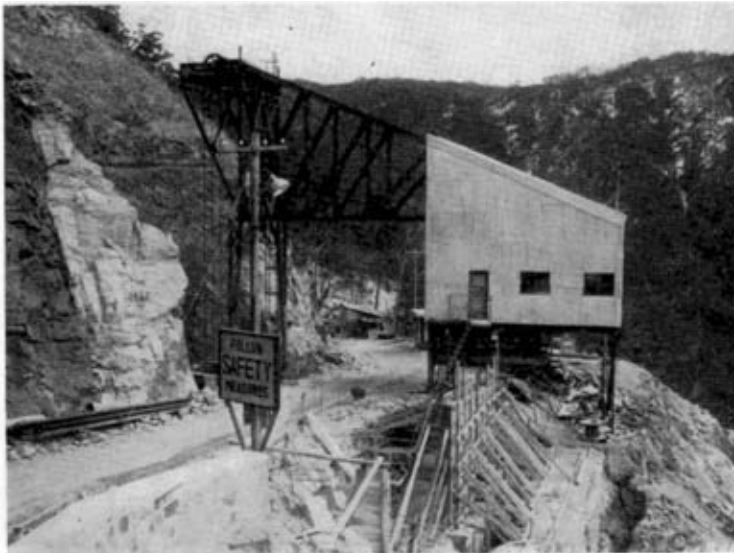
Photo 4. The road down to the power station passing underneath the head frame for Pressure Shaft "A", the top of which is behind the "Safety" notice board. Part of the Lift House retaining wall joined up in foreground.
