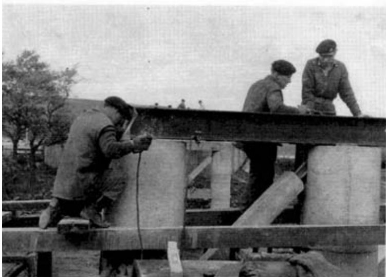
Photo 4. Welding the capsill in position.
