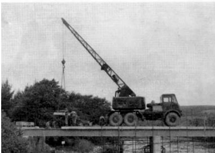
Photo 6. Laying the deck slabs.
