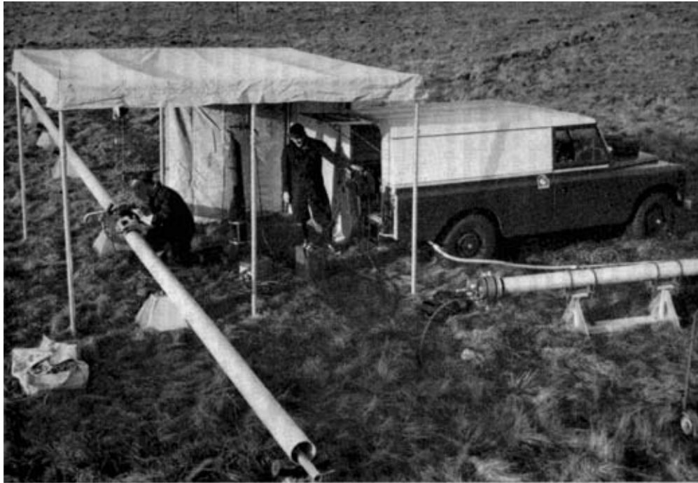
Photo 2. The pipe-welding machine in use in the field, with its generator and ancillary gear on the truck nearby.
