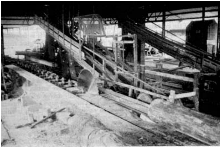
Photo 7. Circular saw and roller table. Electric power mill.
