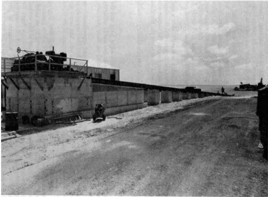
Photo 1. Slipway partially complete showing winch and ramp.
