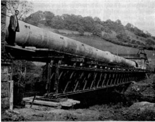
Photo 3. Pipeline resting on Bailey Bridge.
