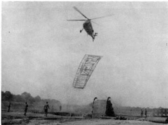
Photo 2. Westland Wessex helicopter carrying the MEXE lightweight bridge to place across the dry gap in the foreground
