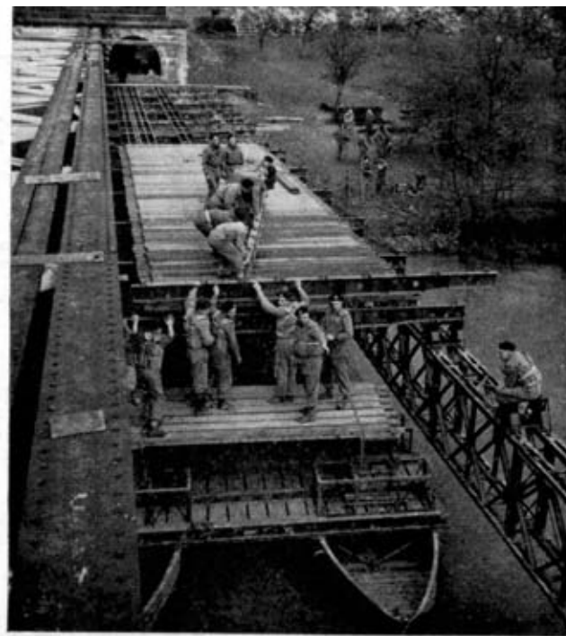
Photo 2. Boat raft, with superstructure used in placing transoms.
