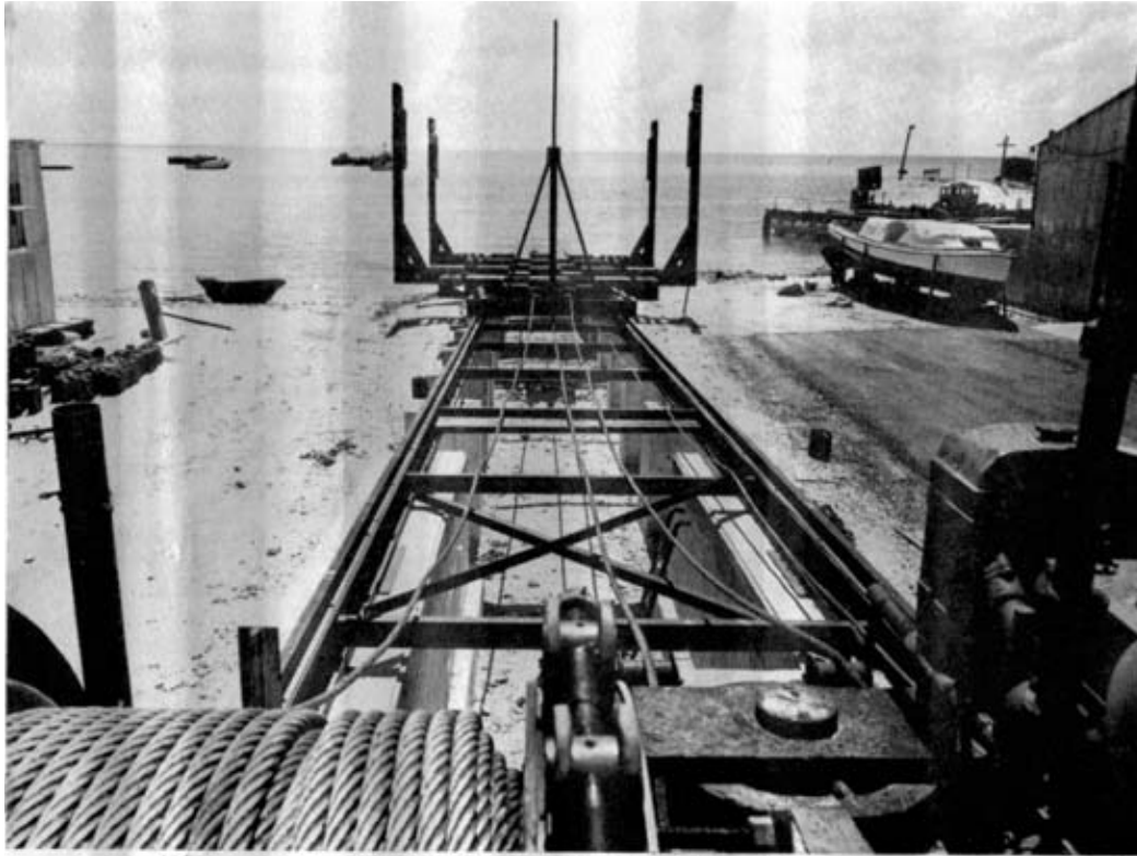
Photo 4. Slipway complete with cradle in position.
