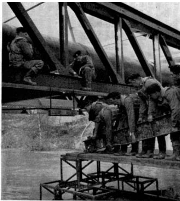
Photo 1. Moving transoms into position.
