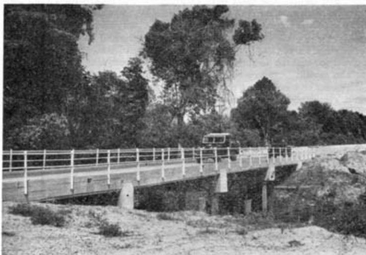
Photo 6. A 137-ft, five-span, prestressed beam bridge on piled piers.
