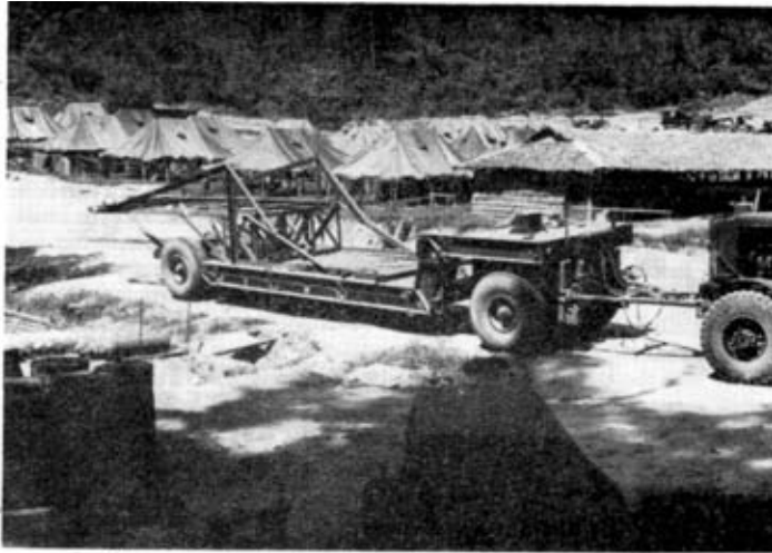
Photo 3. Low loader with platform for 40 ft prestressed RC beams.
