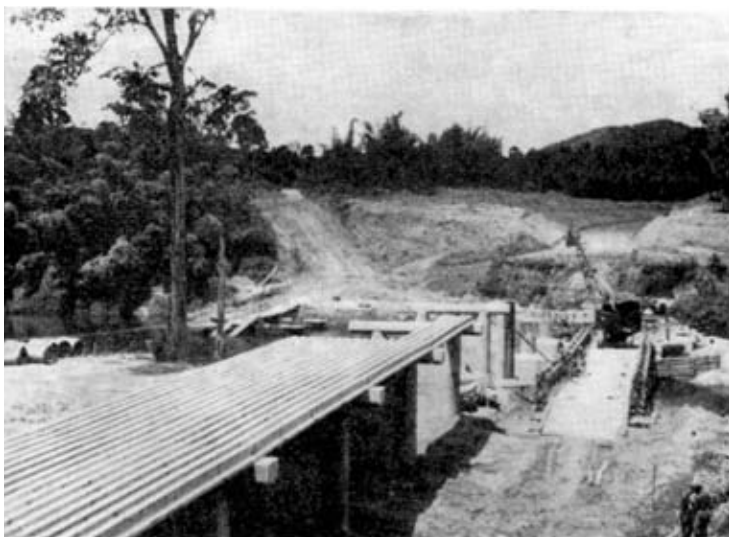
Photo 9. Nami Bridge, deck beams being placed.
