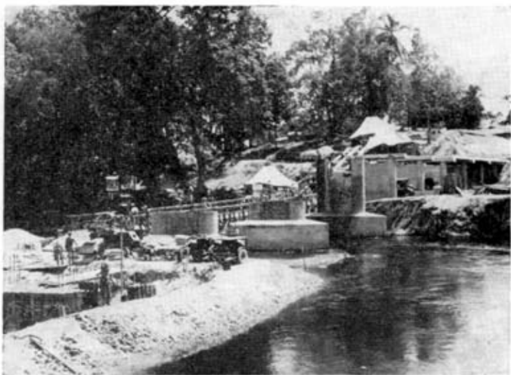
Photo 8. Nami Bridge, river piers under construction.
