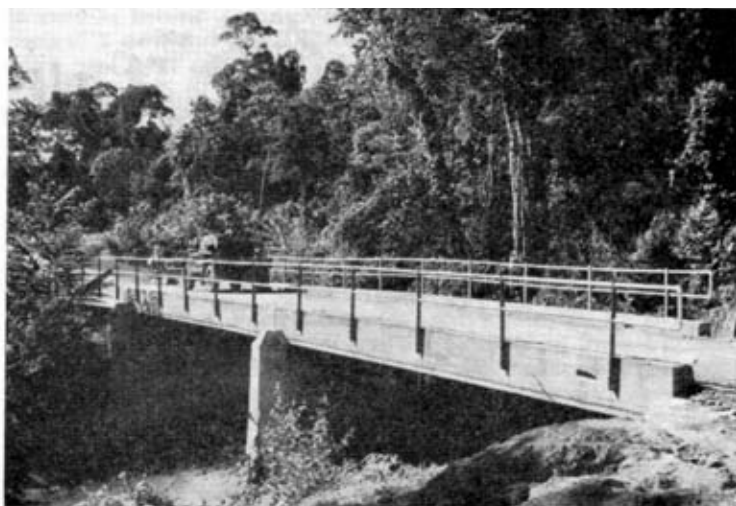
Photo 5. After—a 90-ft, three-span, prestressed beam bridge on mass concrete piers.
