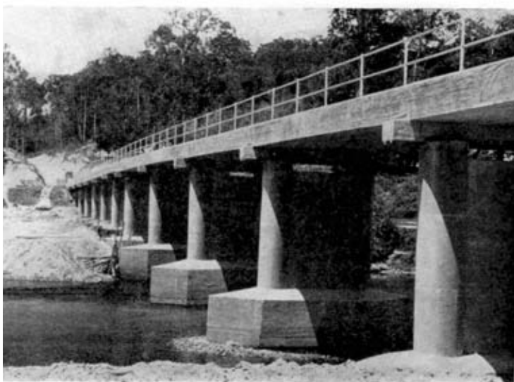
Photo 10. Nami Bridge, showing completed piers, before cement-wash treatment.
