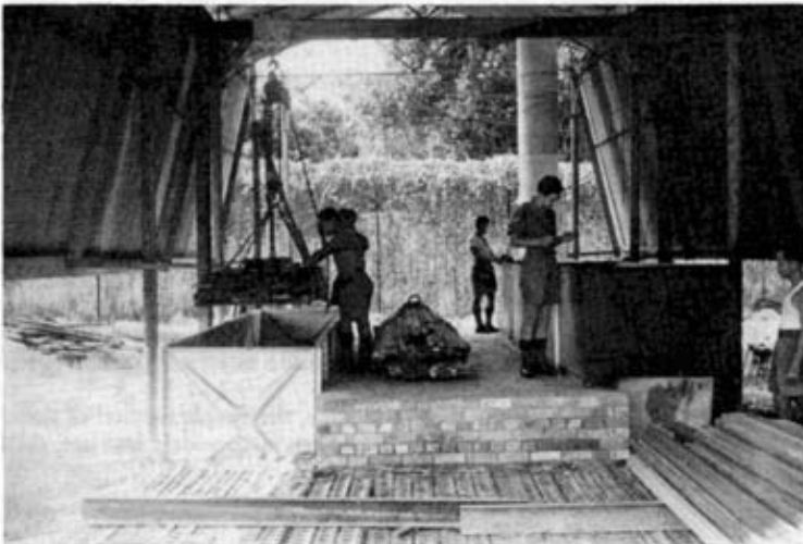
Photo 4. Detail of "hot" and "cold" tanks. "D-B" treatment plant.
