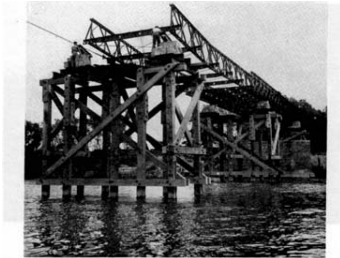
Plate 2. The nose of the bridge reaching the final pier, details of which are clearly shown. The remains of the eastern stone pier will be just submerged under flood conditions.
