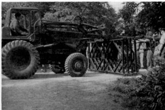
Plate 5. The light-wheeled tractor delivering a load of panels to the construction site.
