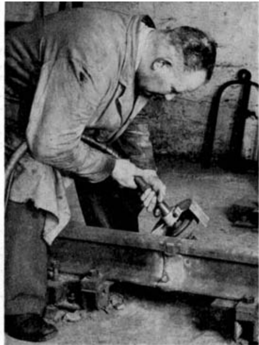
Fig 14. Hand grinding running edge, 109 lb/yd rails.
