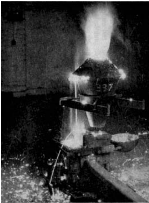
Fig 13. Thermite reaction 109 lb/yd rails
