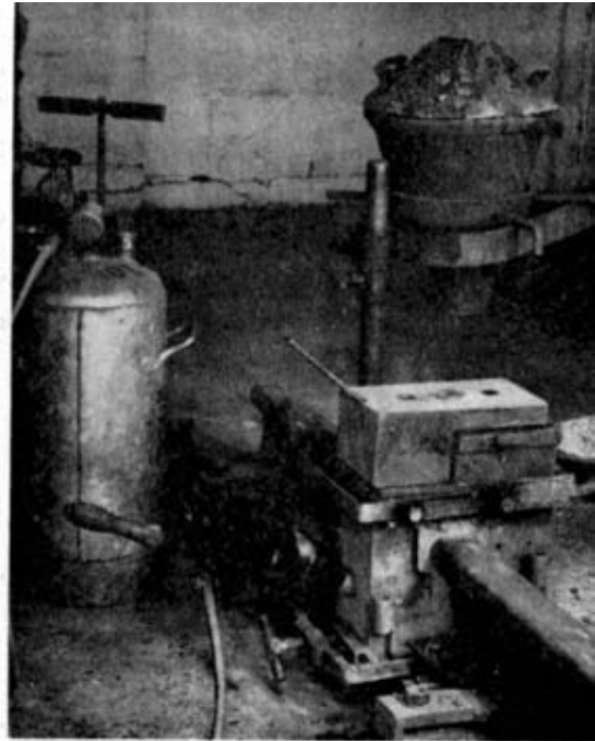
Fig 12. Preheating crucible charged and ready to swing into position for pair 109 lb/yd rails
