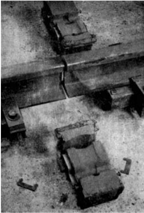
Fig 11. Rails set for welding 109 lb/yd rails
