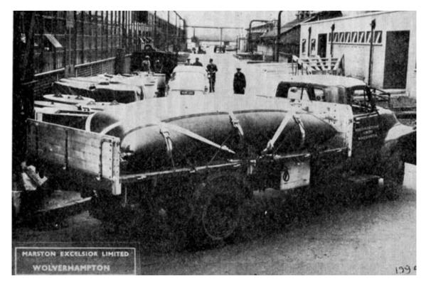
The use of modern flexible containers in water supply 1
