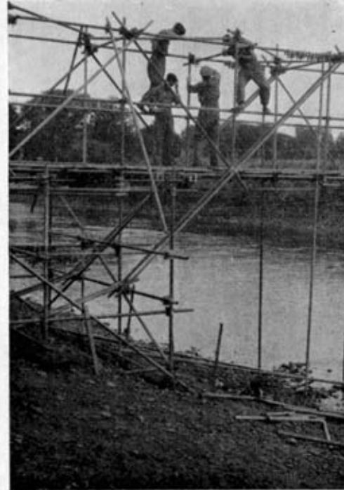
Photo 3. —Work in progress on home bank, showing doubled diagonal struts
