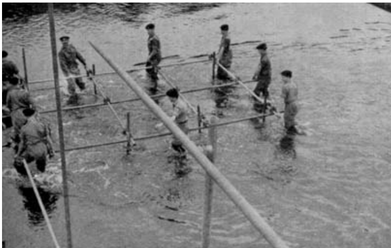
Photo 1. —Placing one of the pier bases.
