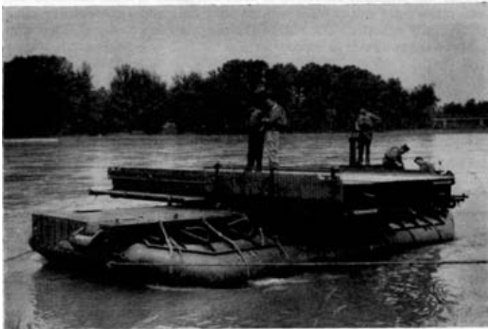
Photo 3. —The Deck unit afloat with the decking swung into the line of bridge.
