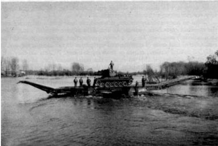
Photo 10. —A Patton tank on a Class 30 raft. The raft commander is standing on the tank turret.
