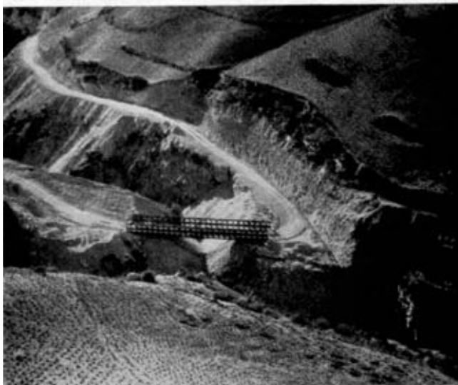
Photo 2. An aerial view of the far bank approaches, showing the cliff which had to be cut down.
