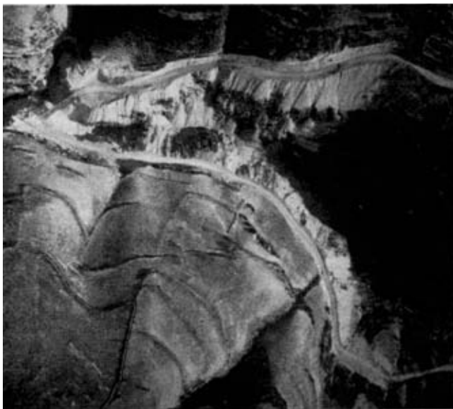
Photo 1. A view of the majority of the road work. The light area is all fill from road excavation.
