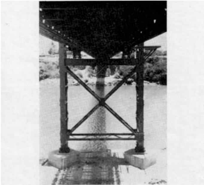
Photo 2. Showing rocker bearings.
