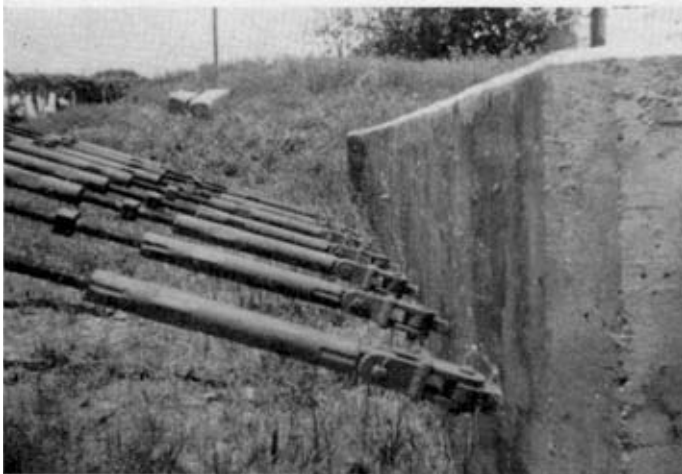
Photo 3. Showing steel line anchor ropes.
