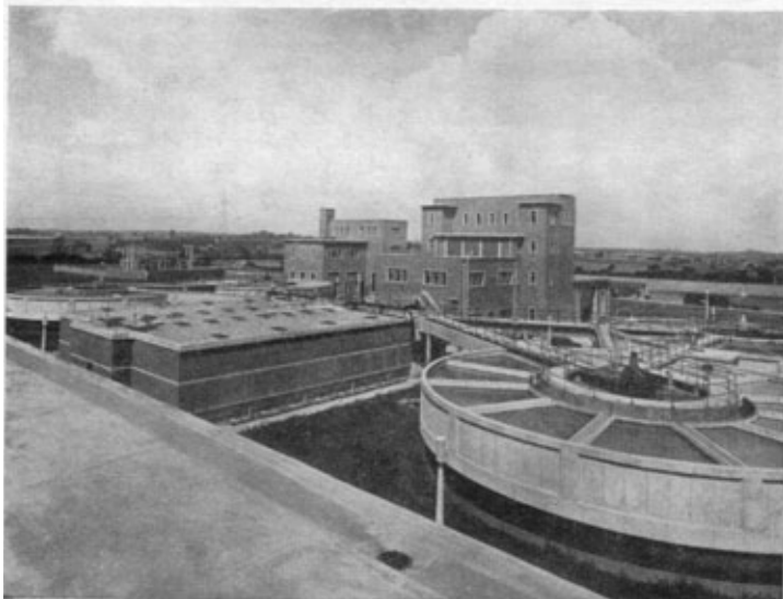
Photo 2. —The Treatment Works. A view from the roof of the Filter House showing the circular Accelerators, the Contact tank in the foreground and the Chemical and Boiler houses. The electricity sub-station can also be seen.
