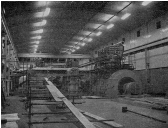
Photo 1. —General view of Power Station showing three General Electric 1,000 kW. sets and the gas turbine under construction.
