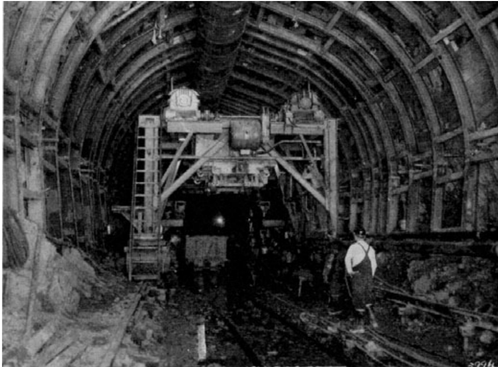
Photo 3. —Eucumbene-Tumut tunnel, "Cherry-picker" in operation.
