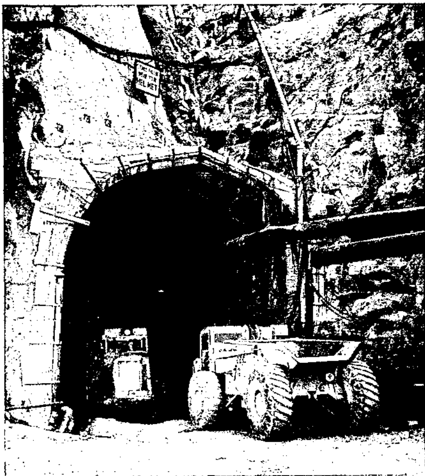
Photo 5.—T1 Power Station—Tournarockers in the access tunnel.
