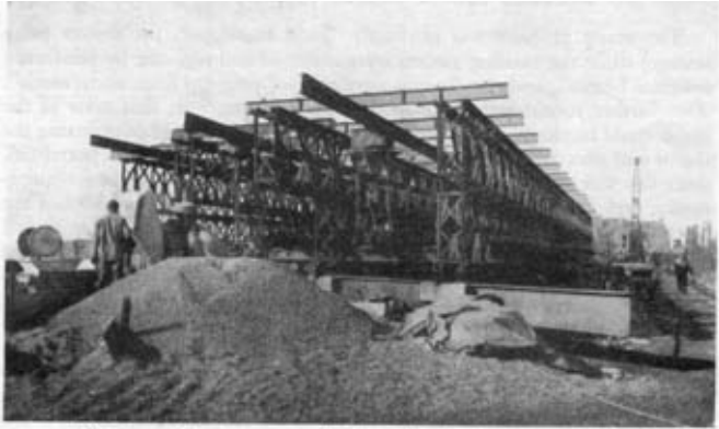
Photo 3. —View from one end of the bridge showing concreting plant.
