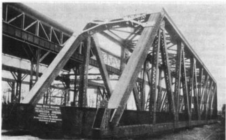
Photo 1. —One of the through spans erected in Poraith Waite's yard. Note drilled plates with eyes at ends of bottom booms.
