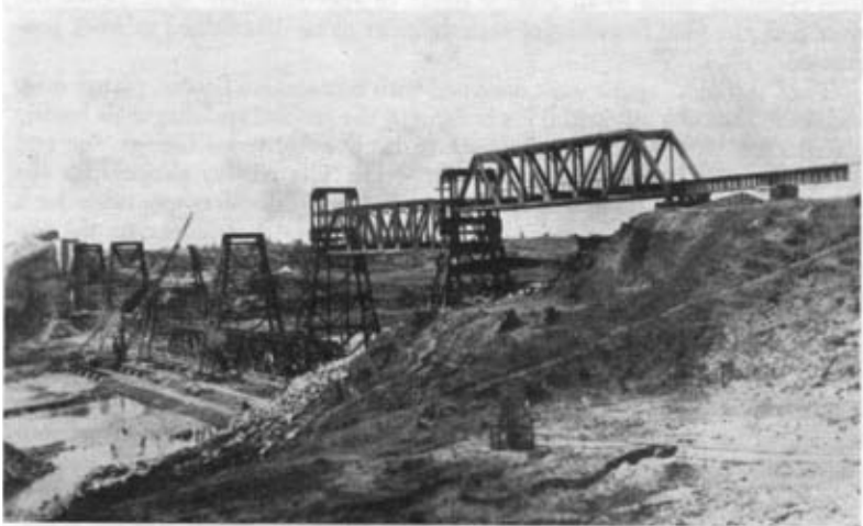
Photo 2. —Through spans being lifted from river bed.
