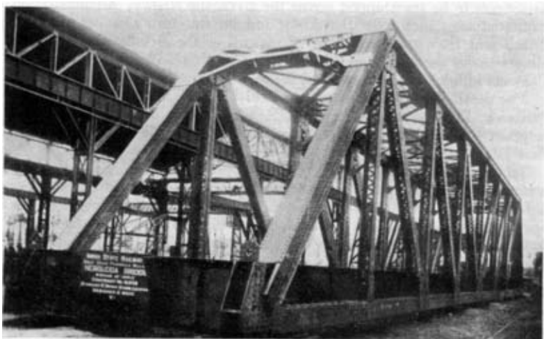
Photo 1. —One of the through spans erected in Poraith Waite's yard. Note drilled plates with eyes at ends of bottom booms.
