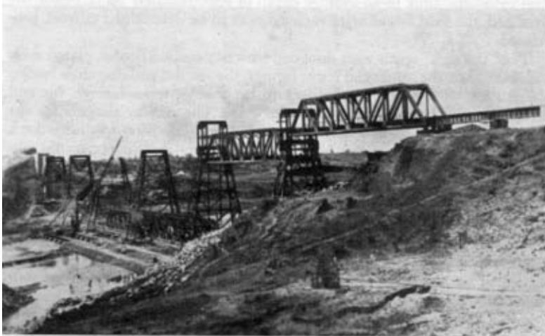
Photo 2. —Through spans being lifted from river bed.
