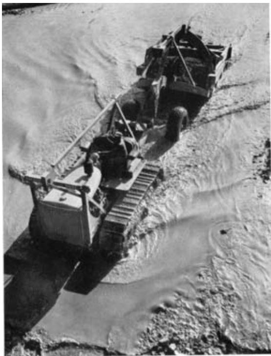
Photo 4. —Caterpillar tractor drawing a scraper to provide fill for approach to a bridge in Korea.
