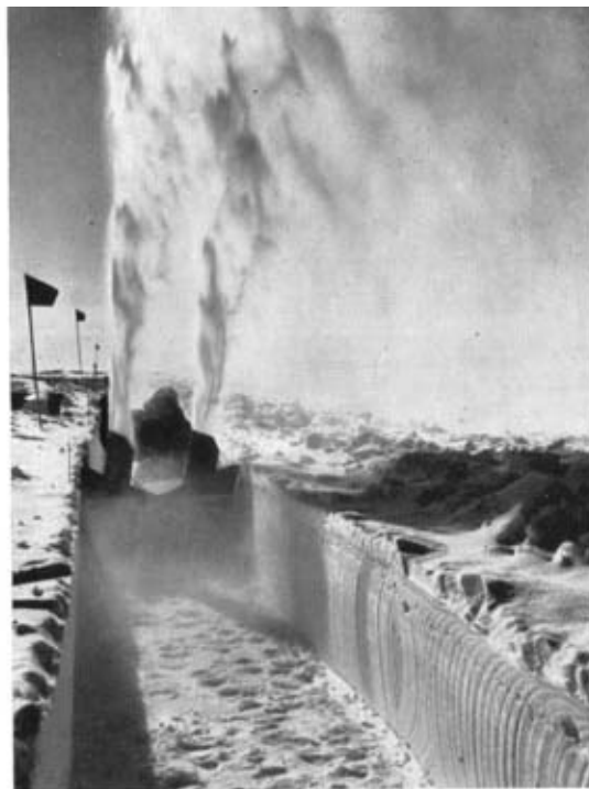
Photo 5. —Four foot trench, eighteen feet deep, being cut in the snow in Greenland.
