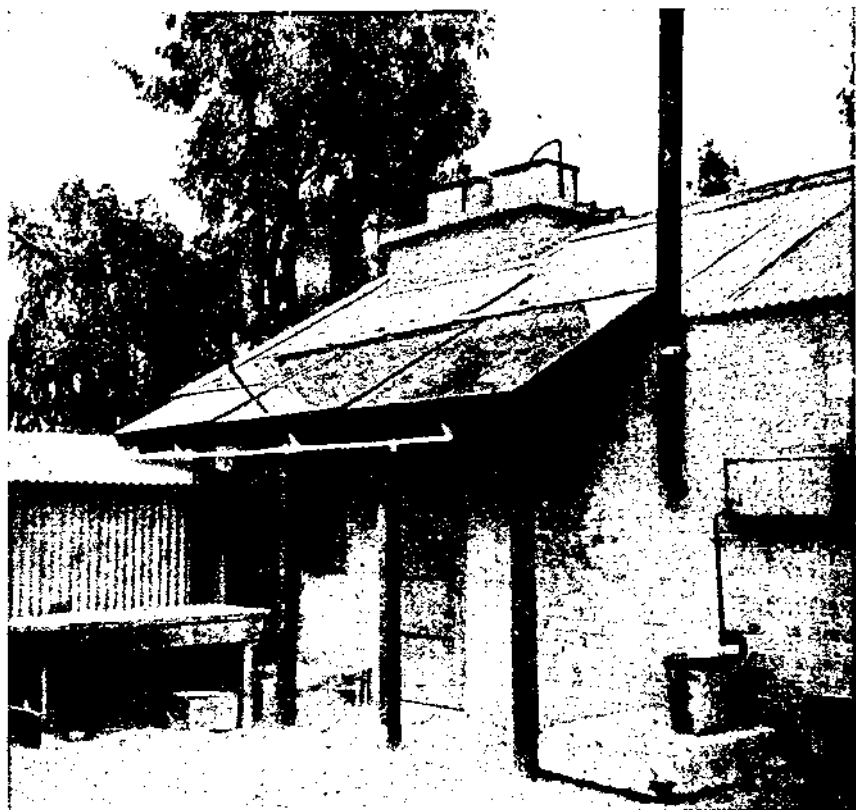
Photo 1. —Solar heater absorber panels on eaves of bath-house. Chimney on right and fuel tank on wall are irrelevant. Header tank on ridge was part of original hot water system, and now serves solar heater.
