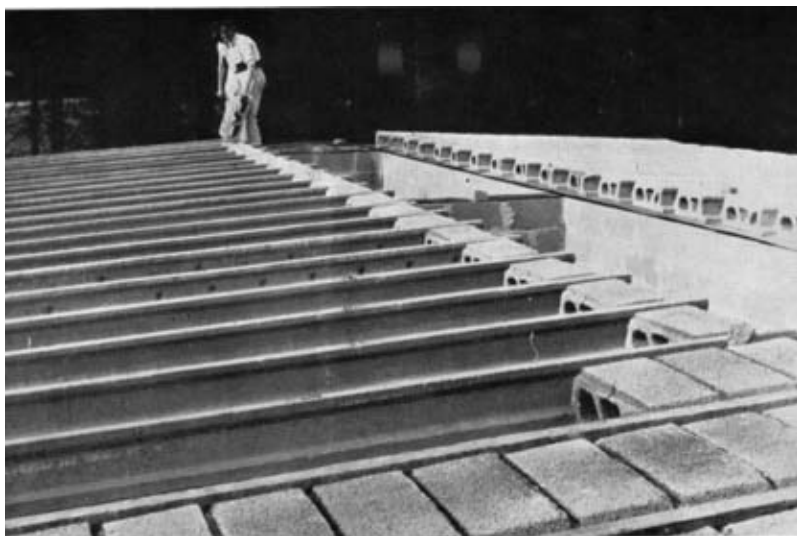
Photo 4. —One of the types of flat roof construction. Its insulation from walls by felt is visible.
