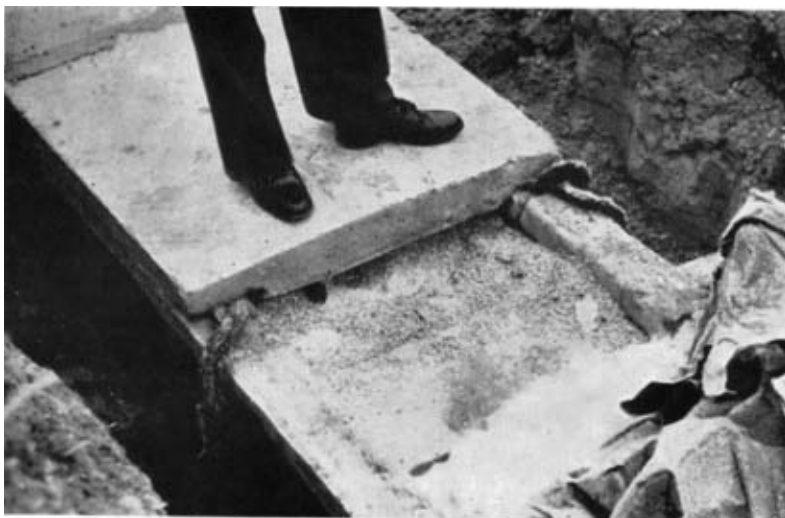
Photo 8. —Heating duct showing concrete cover (with tarred rope seal), and Vermiculite. The glass wool plug is to contain the vermiculite at a point of change.
