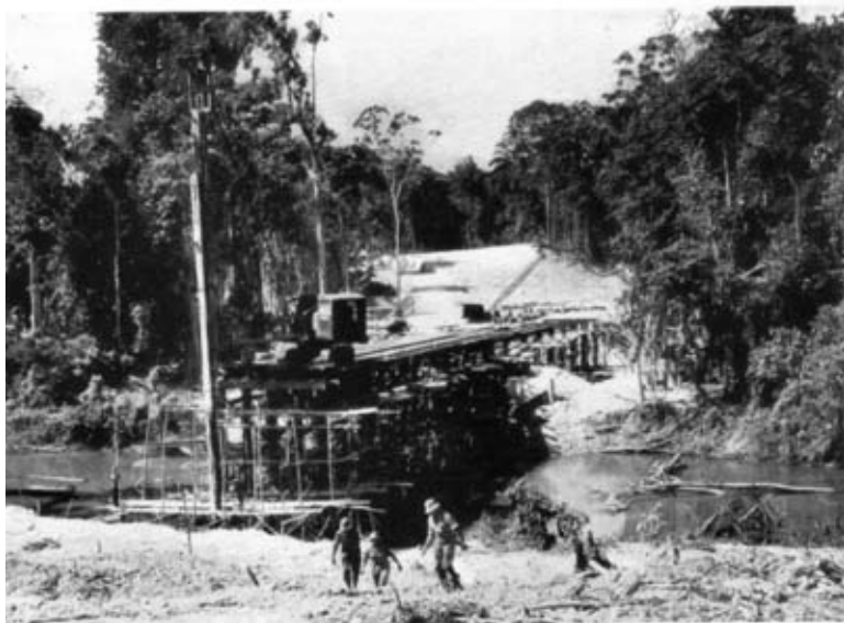
Photo 4. A pile in Bent 16, having been placed, is being adjusted prior to driving. In the background a 19 R.B. crane is working in the stores site.
