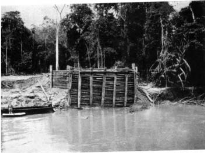
Photo 1. Retaining wall on south bank seen from the north bank. The cracked pile can be seen on the right of the picture. The restraining cable passes over a back baulk of timber about two feet below the tops of the piles.
