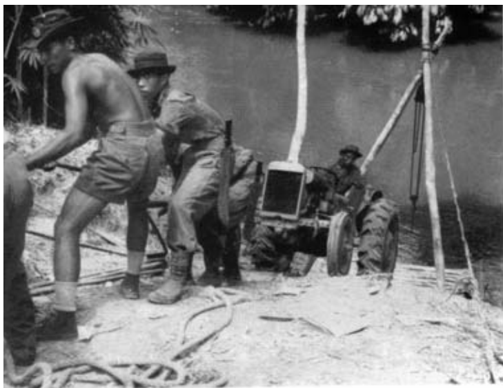
Photo 1. —Fort Dixon Airstrip. A Ferguson tractor brought by boats in pieces has been assembled and is being hauled up the river bank by Malayan Sappers.
