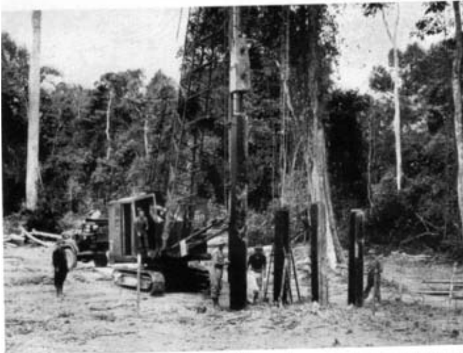
Photo 2. Pile driving in Bent 2. The pile driver tracks are parallel to the line of bridge. A bent lifting bolt can be seen at the top of the left-hand pile.
