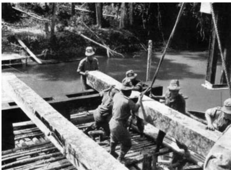
Photo 3. Placing a roadbearer. The pile driver is being used to lift the road bearer.
