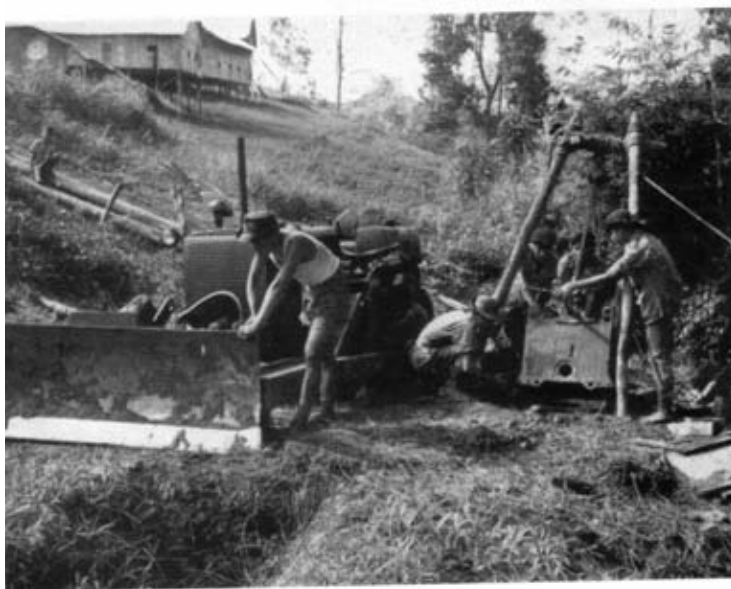
Photo 2. —Fort Dixon Airstrip. A Size IV tractor, brought to site in boat loads, being assembled.
