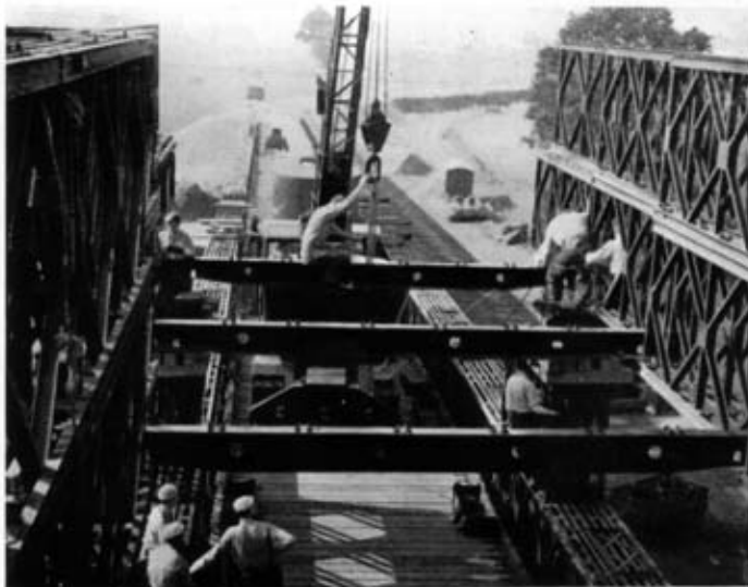
Photo 8. —The tail of the navigation span being constructed.
