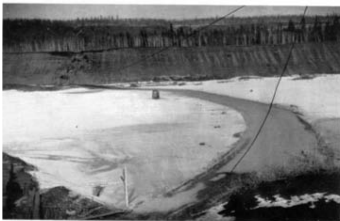
Photo 4. —Ice bridge at Pelly River. General view looking north (note damp roadway) Bridge length 230 yds.
