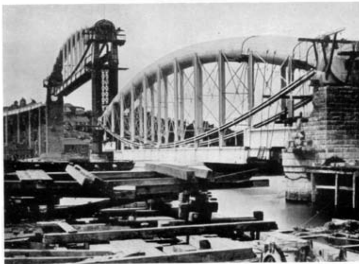
Photo 4. —Saltash Bridge. Raising the girders from pontoons.
