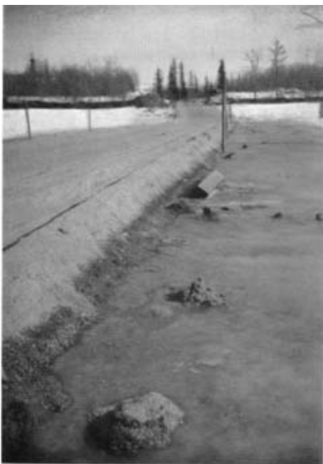
Photo 3. —Ice Bridge at Yukon River. Detail of raised carriageway and sawdust covering.
