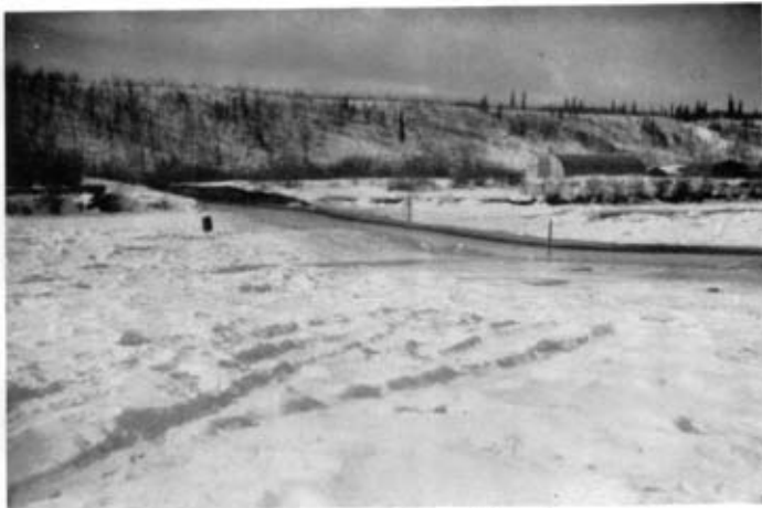
Photo 2. —Southern bank showing ramped down ice approach.
