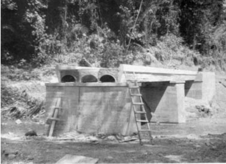
Photo 3. —Dry Creek Bridge under construction showing jack-arch design.
