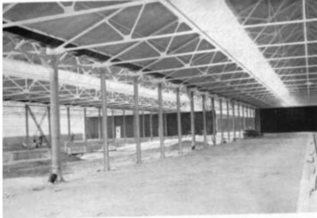
Photo 3. —General view across bays in Shed 3 with central drainage channel and under floor drainage being laid, near bay covered with gravel but with no floor laid.
