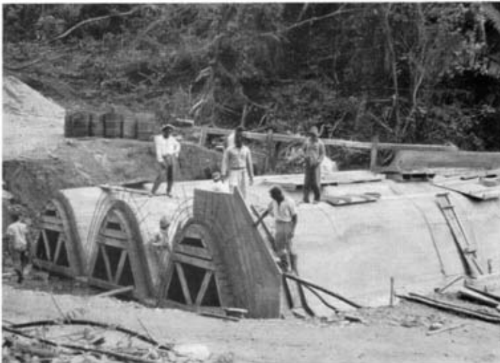
Photo 4. —Triple parabolic culvert under construction, showing shuttering for headwalls being erected.
