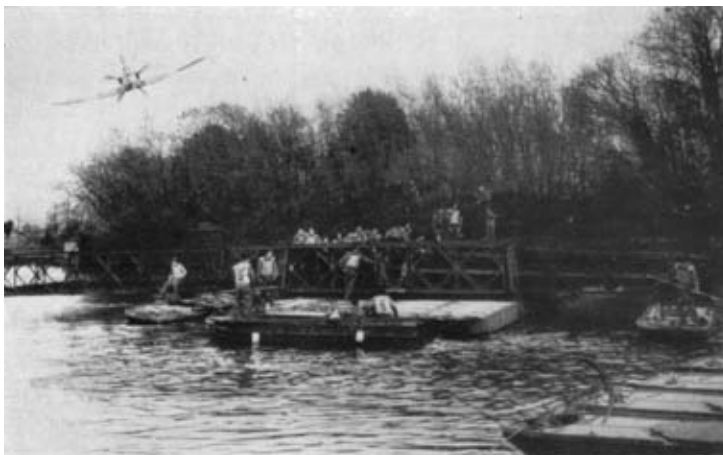
Photo 1. —Landing bay on landing bay raft ferried across to the far bank.
