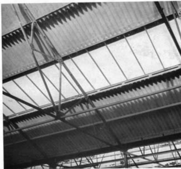
Photo 4. —Detail of underside of roof, glazing and sheeting complete.
