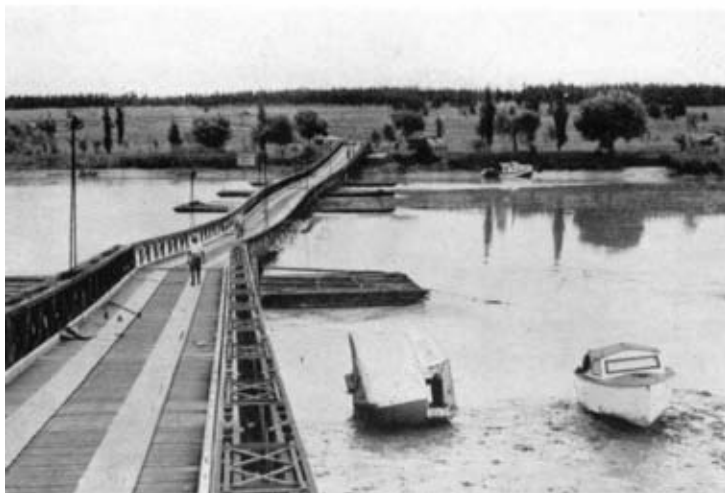
Photo 2. —After one landing bay had been pulled into alignment. The low portion where the pontoon piers had been lost is clearly visible, as well as some of the boats saved.
