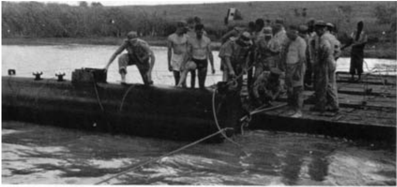
Photo 3. —Keeping the steel pipe away from the pontoons to avoid damage.
