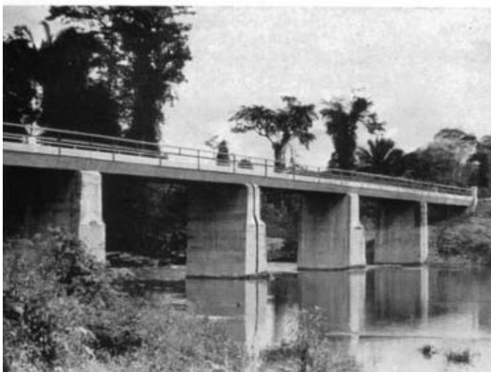
Photo 2. —Caves Branch Bridge. Six spans of 44 ft. steel girders and jack-arch deck.
