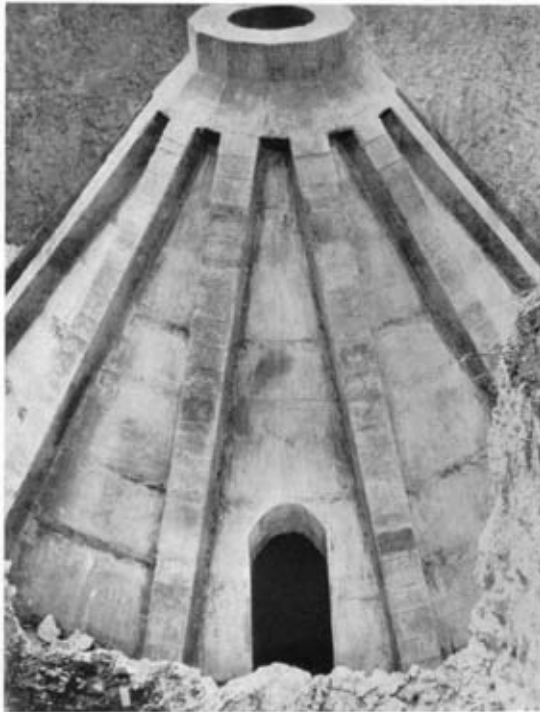
Photo 6. —Soakaway cap, R.C. work complete.
