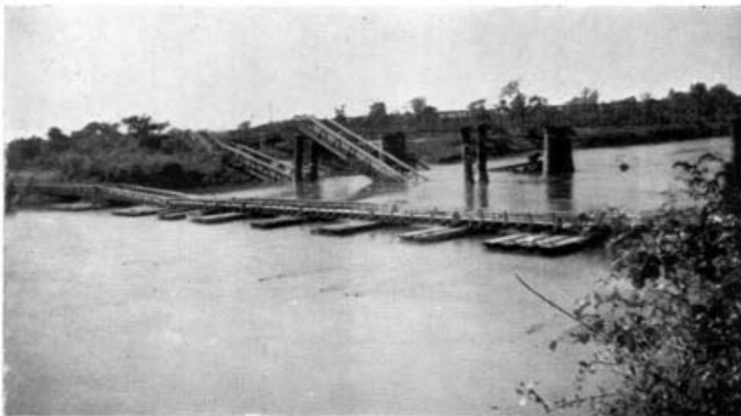
Photo 2. —Site "Y" January, 1946. The diversion pontoon road bridge, with the continuous Bailey at Site "Z" 200 yards downstream.
