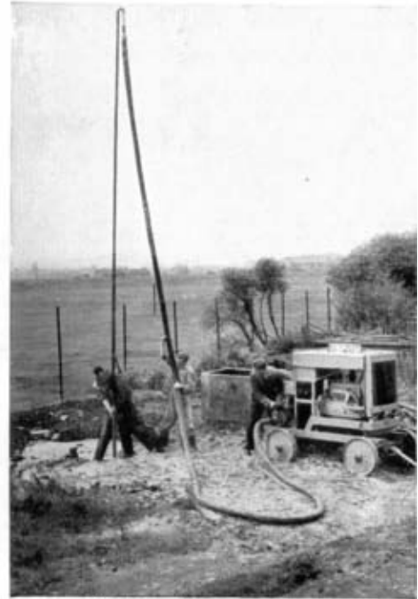
Photo 2. —Jetting in a well point.
