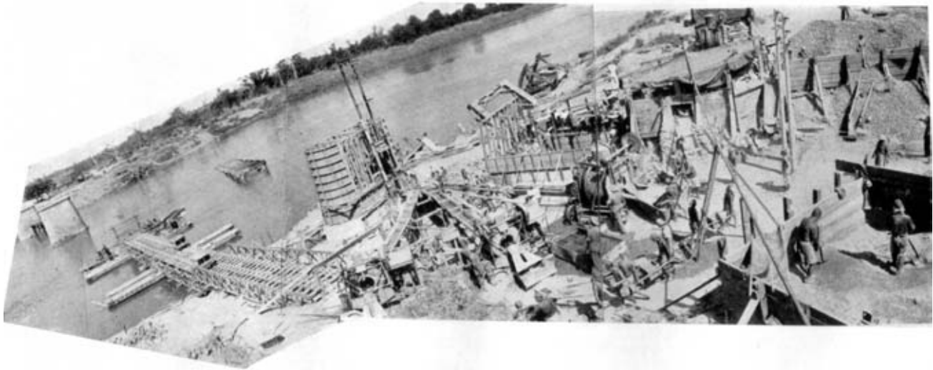
Photo 3. —Site "Z" April, 1946. Concreting in progress at No. 5 pier. Construction bridge laid to stump of No. 4 pier.
