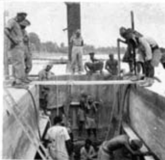
Photo 5. —The anti-flood rim, showing Indian Sappers and Miners working alongside J.S.Ps.
