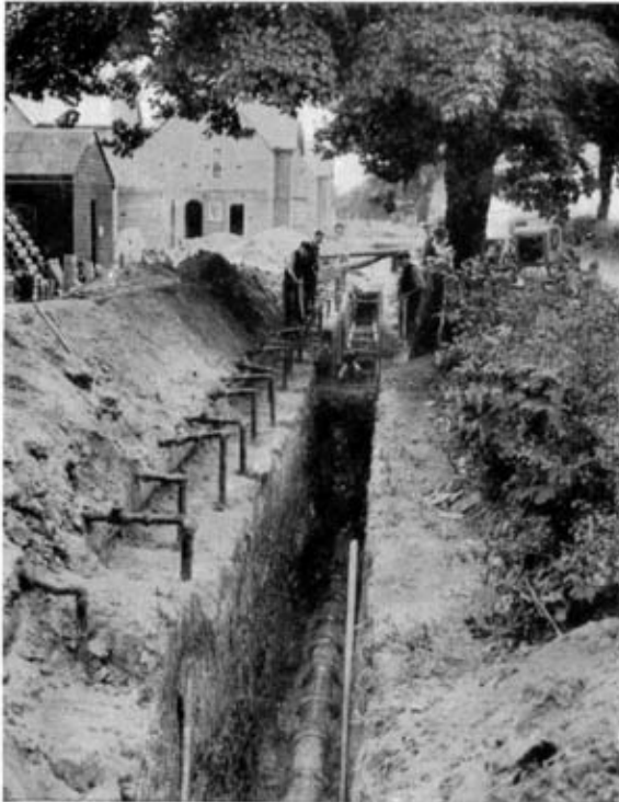
Photo 1. —A trench excavated 11 feet deep in heavily water-logged ground after dewatering by means of the line of well points shown on the left of the trench.
