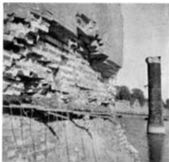
Photo 4. —Pier No. 4. Decapitation by Beehive charges. Ready for the second blow.
