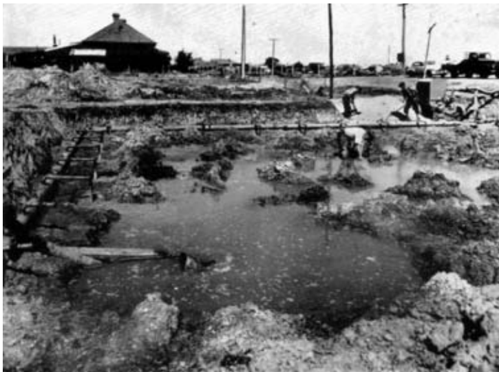
Photo 3. —Permanent water level on a site in South Australia before dewatering.
