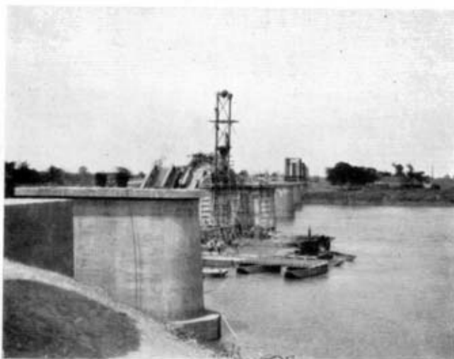
Photo 6. —Site "Z" June, 1946. Pier No. 4 nearing completion, and the new Warren girder span ready for launching on the south bank.
