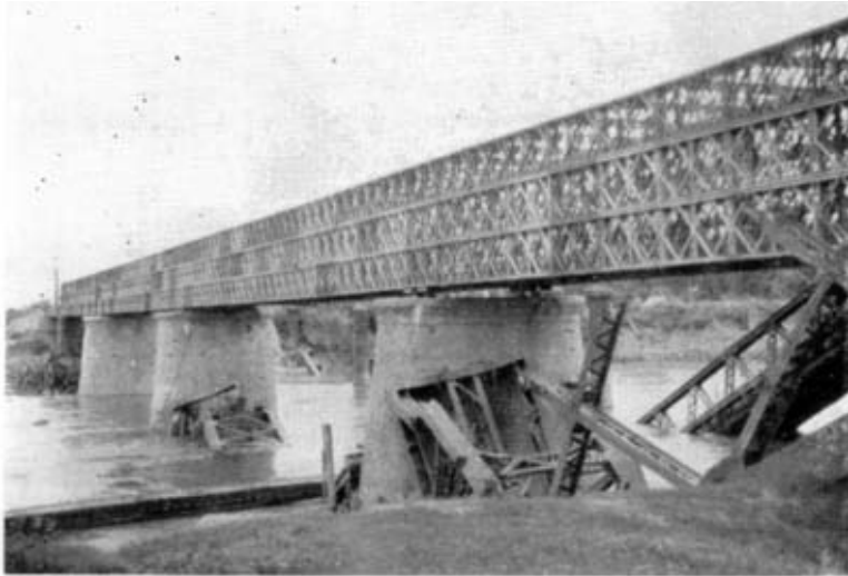
Photo 1. —Site "Z", December, 1945. The 830 ft. temporary Bailey bridge, showing original brick piers and wreckage of pre-war Warren girders.
