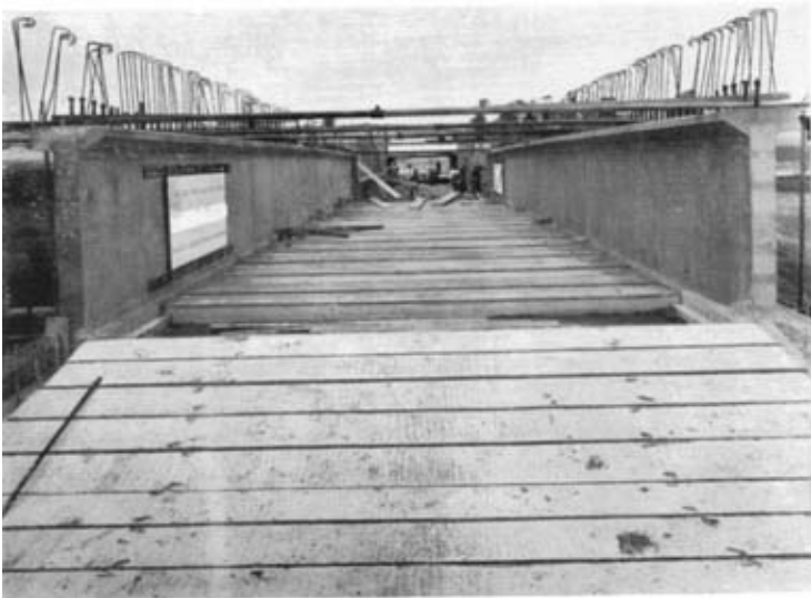
Photo 4. —The lower deck of the bridge under construction. The post-tensioning of the main girders is complete and the precast hollow units of the lower deck can be seen in position in the foreground.
