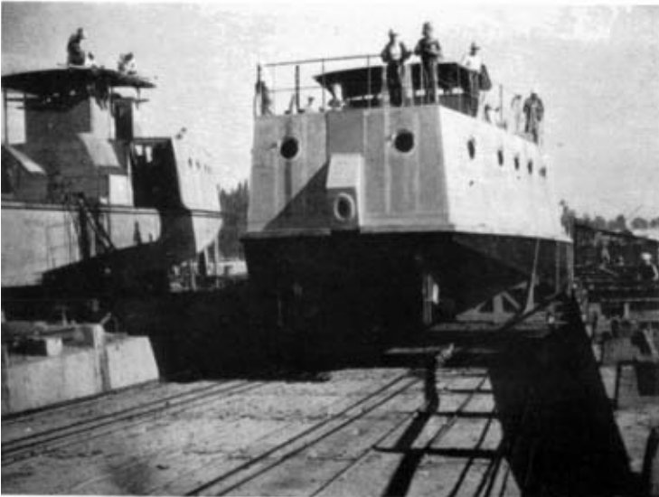
Photo 4. —Z Craft (Type B) on cradle. Note difference between sterns of Type A and Type B.
