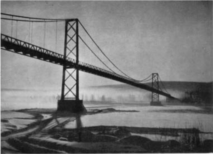
Photo 3. —The Peace River bridge. Bagged concrete is being dumped through the ice around the pier to prevent further scour.
