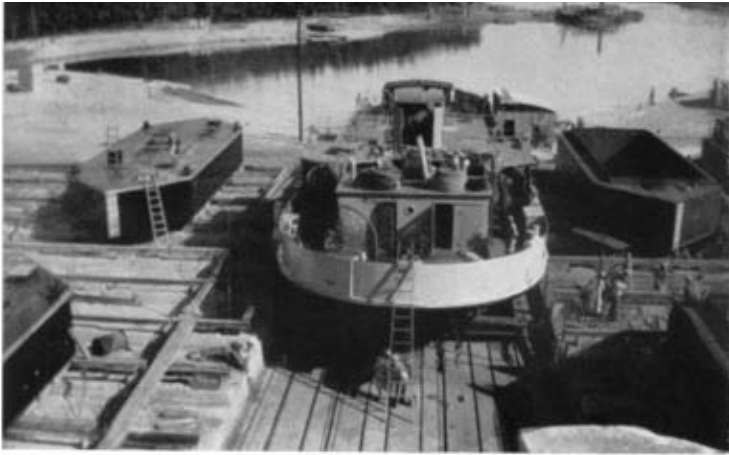
Photo 3. —Z Craft (Type A) on cradle and dumb barges on stocks.
