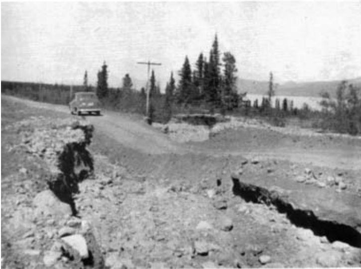
Photo 2. —Temporary fill over a washed-out culvert.
