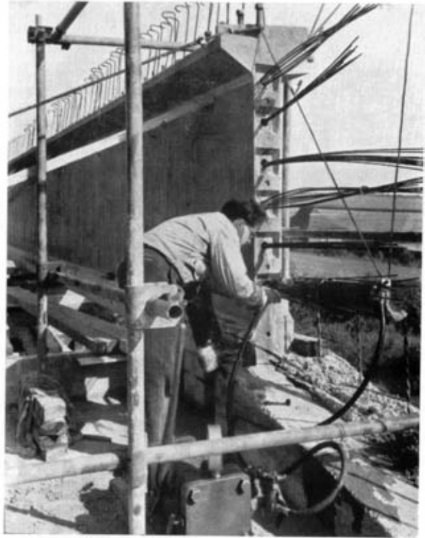
Photo 2.—Stressing one of the main girders.
