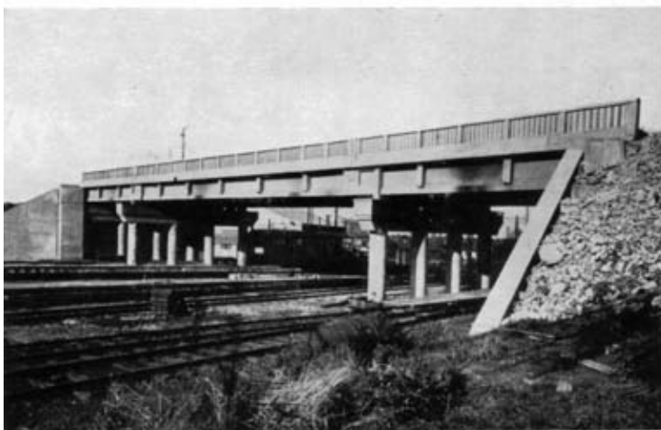
Figure 2. —Lille bridge, completed, showing tell-tale ribs concealing transverse prestressing anchorages.
