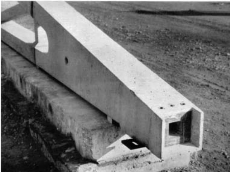
Photo 2. —End anchorage block of a roof truss.
