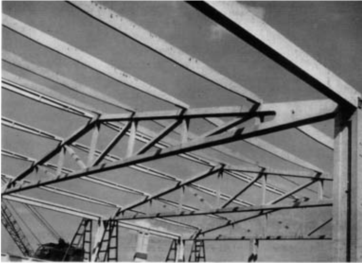
Photo 1. —Roof trusses and purlins in position.
