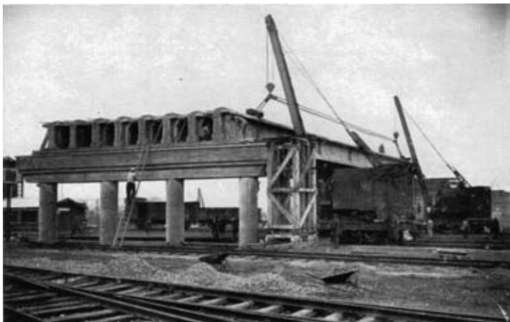
Figure 1. —A road-over-railway bridge at Lille under construction, showing the characteristic bottom flanges of the beams.
