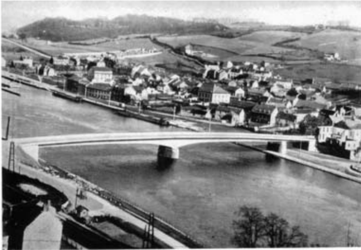
Figure 3. —Bridge at Sclayn, Belgium. Typical example of continuous beam construction, with beams tapering towards the abutments.
