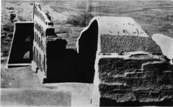
Photo 1. —The Great Arch of Ctesiphon. The ancient Persians built this of Tigris mud. They got the shape right. That is why it has been able to withstand the centuries.
