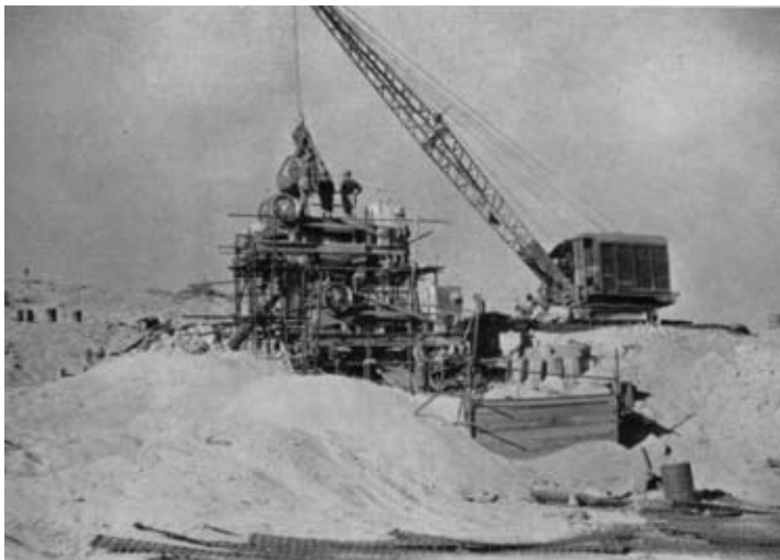
Photo 6. —Rock crushing plant.
