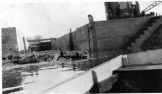
Photo 3. —The Sapper task nearing completion. Concreting work finished, the piles extracted and all that remains to be done, is the removal of the debris which was in front of the downstream piles. This can be seen in the foreground of the photo.
