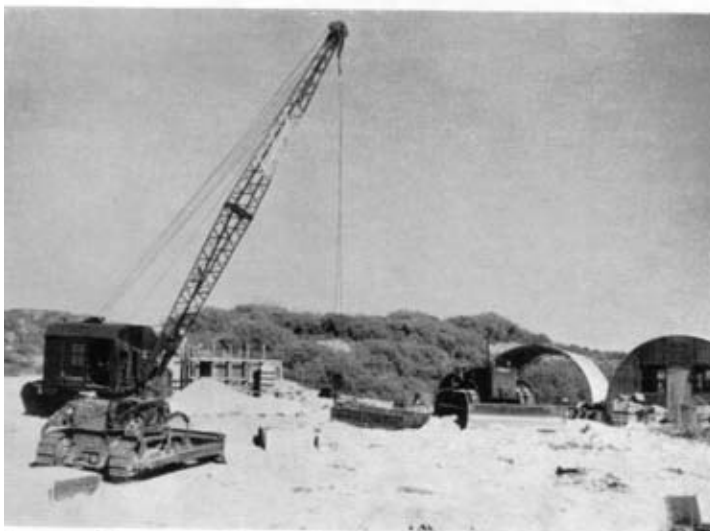
Photo 7. —19 R.B. crane showing repairs to jib in light colour. This photo also shows a bulldozer and sledge and some Nissen huts in course of construction.
