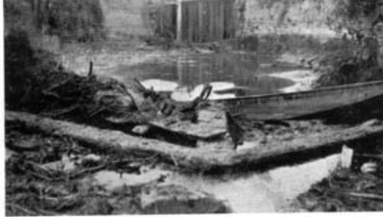
Photo 1. —Dewatering completed showing original state of lock bottom and badly cracked, bulging walls.
