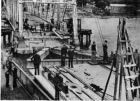
Photo 2.—View of the three-leg link of welded plate girder design.
