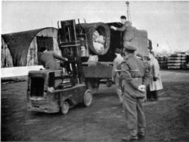
Fig. 7. —Clark 6,000-lb. capacity depot type forklift truck with solid tyres loading barbed wire parcel into a covered 3-ton lorry from the rear.
