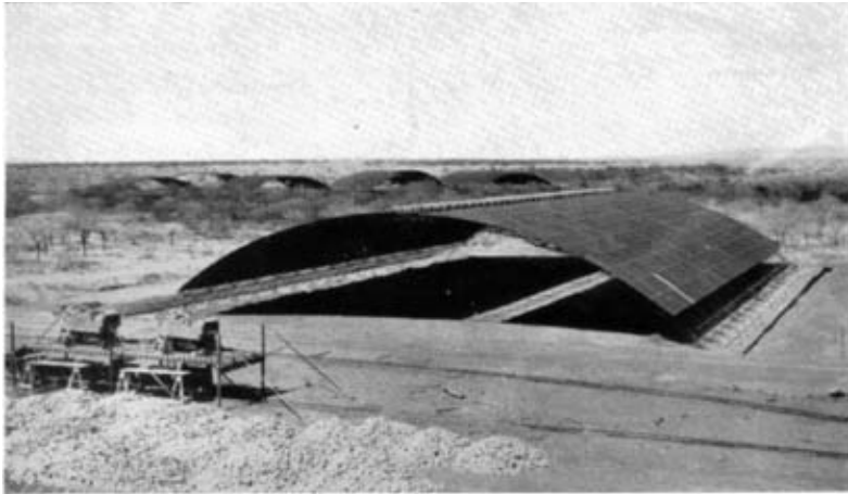
Photo 5.—“ Igloo ” partially clad.
