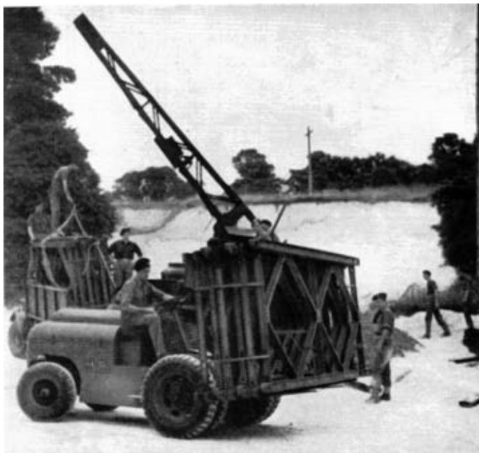
Fig. 3.—3-ton Coles Crane and “Matbro” forklift truck working together on the unloading and delivery of parcelled bridging stores to a bridging site.
