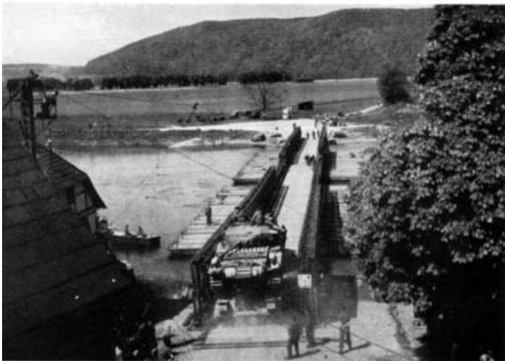
Photos 3 and 4.—Class 80 B.P.B. with Tank and transporter crossing it.
