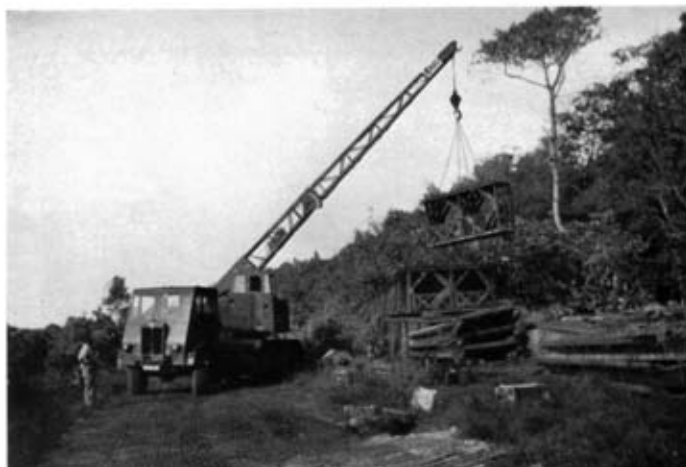
Fig. 4.—7-ton Bridging Crane handling panel parcels in C.M.A. for Exercise “Surprise Packet.” Note length of jib and general handling capacity of this crane.
