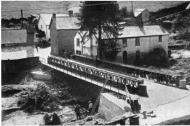
A general view of the bridge at Barbrook in which the work done to the abutments can be seen. Note the " high-water mark " on the white cottages.
