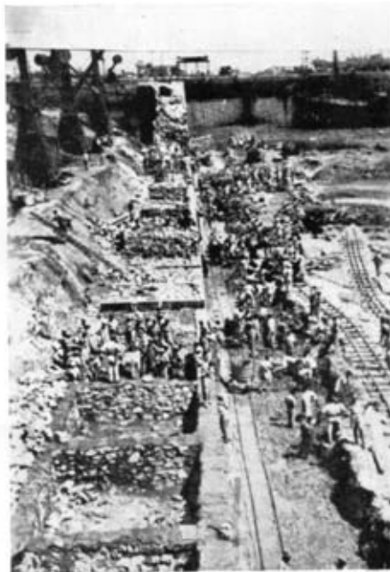
Photo. 4. —Rebuilding north quay wall.
