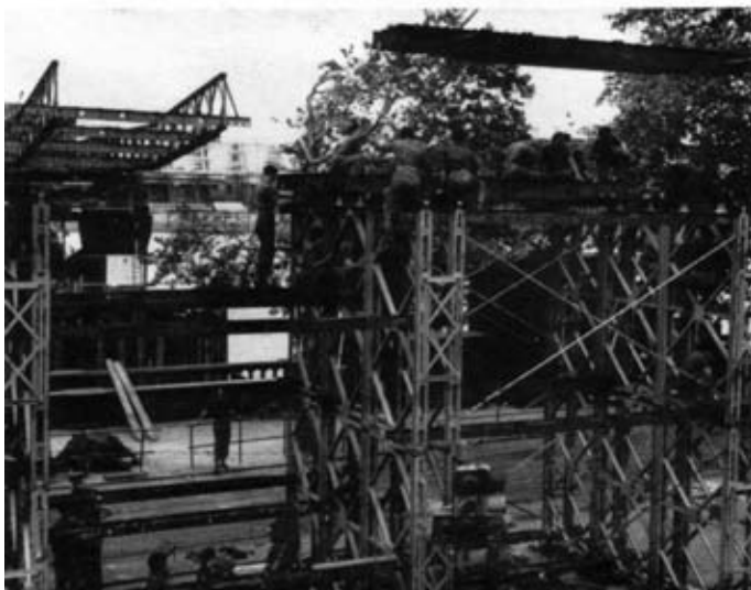
Photo 5.—Erecting temporary pier on North Bank. (Crown copyright reserved)
