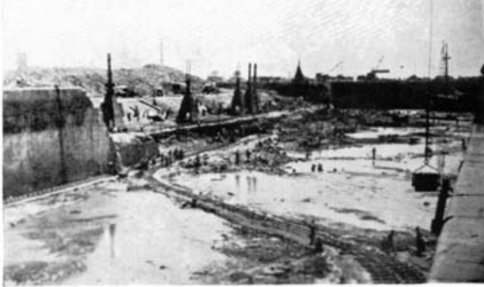
Photo 3. —Initial clearance of shattered north quay wall.
