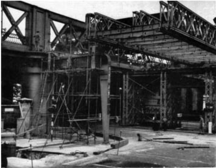
Photo 2. —Portal Frame on North Bank. The white line in the foreground indicates boundary of District Line Tube from Charing Cross towards Westminster. (Crown copyright reserved)
