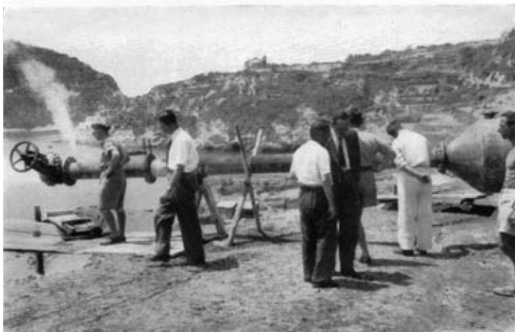
Photo 2. —Steam jet from capped bore at San Angelo.
