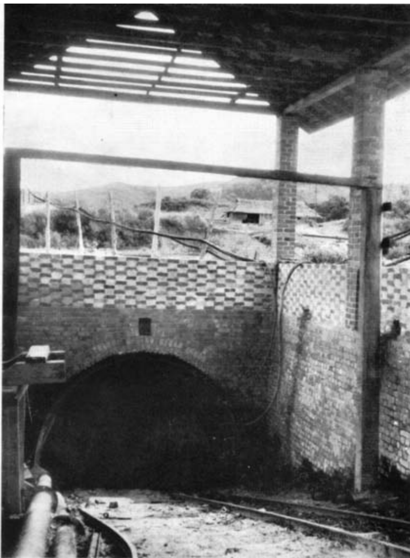
Photo. 1. —One of the main shafts inclined at a dip of 1 in 4. On the left are the delivery pipes of the pumping sets. On the right is the trolley line up which are hauled the tubs of coal
