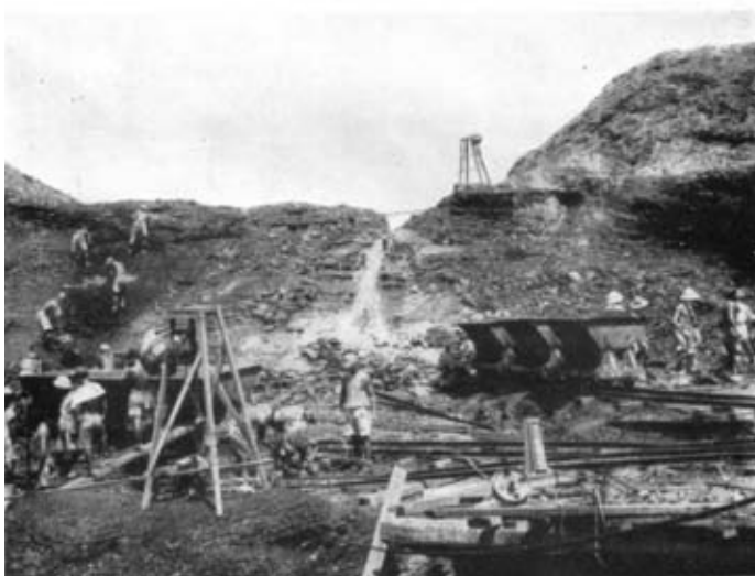
Photo 3. —J.S.P.s. quarrying coal at an open-cast seam. The improvised lighting system made night work possible.
