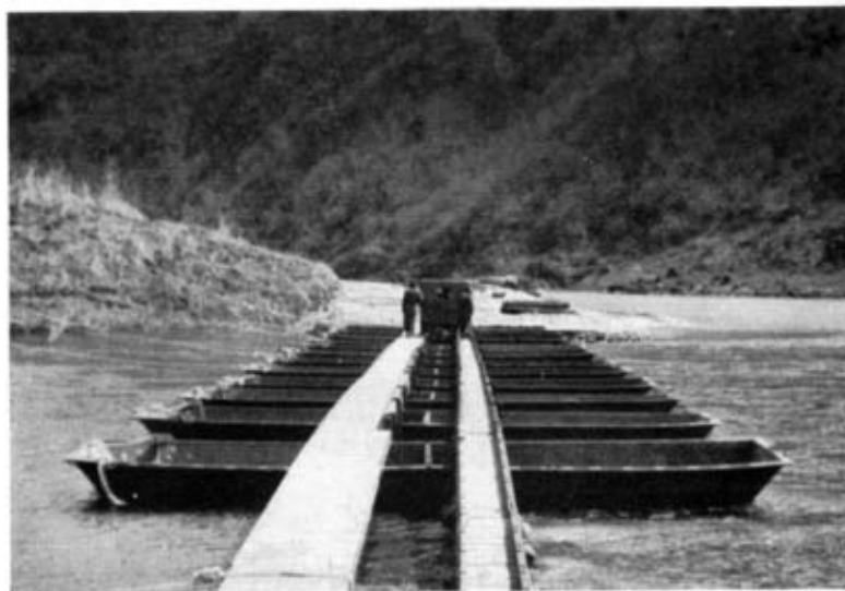
Photo 6. —Afternoon 11th April. Semi-improvised bridge across Imjin river. Note footbridge decking upside down on downstream side of bridge.
