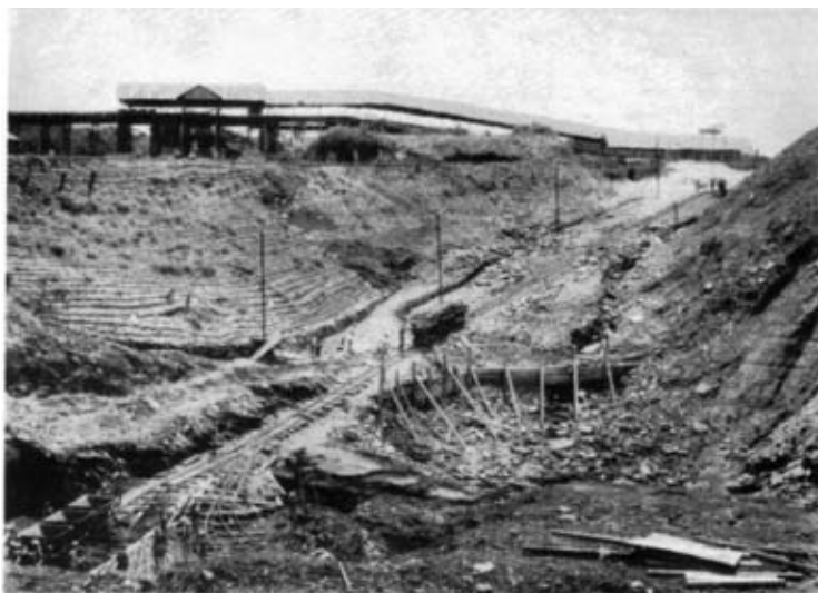
Photo 4. —A general view of an open-cast pit, showing “ skips ” being hauled up towards the “ hoppers ” at left background.
