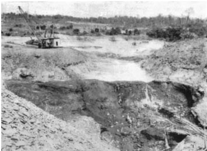
Photo 2. —The bared coal seam. Here J.S.P.s. are loading "skips" by hand. In the right background a dozer is removing overburden. At the left is a giant derelict excavator ruined by the Japs.
