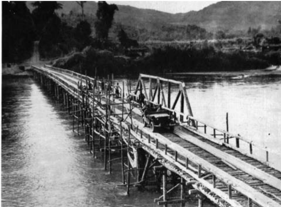
550-ft. piled bridge over the Bilin river built by Japanese, under supervision of 60th Indian Field Company, between Bilin and Papun. This bridge carried Class 12 traffic. All timber was extracted locally. The wide span under construction was for the passage of logs.
