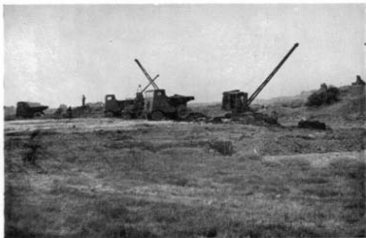
Photo 2. —Excavation from hard roads. Loading 6 cu. yd. dumpers.
