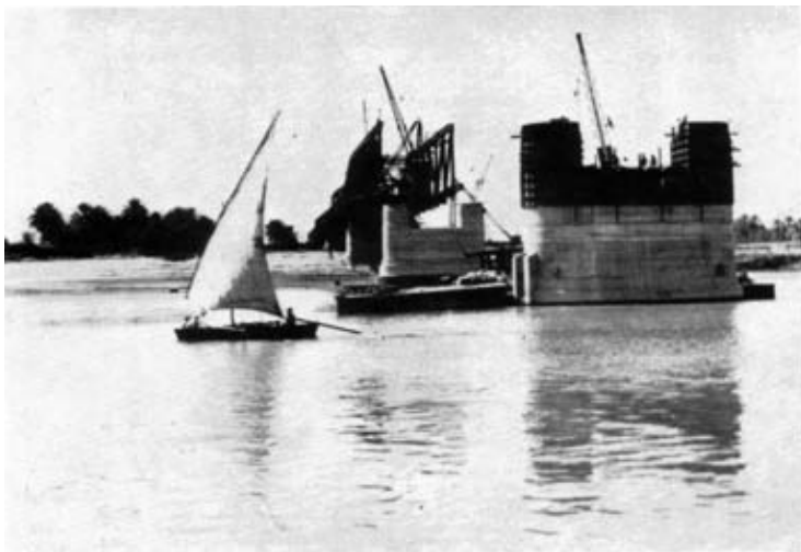
Photo 4. —River pier under construction showing climbing steel shuttering.
