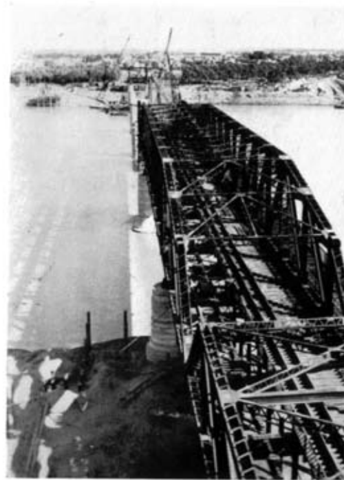
Photo 7. —Overhead view of bridge, showing stringers on left ready to take railway ; roadway in centre with temporary rail track for construction purposes ; and footpath on right.
