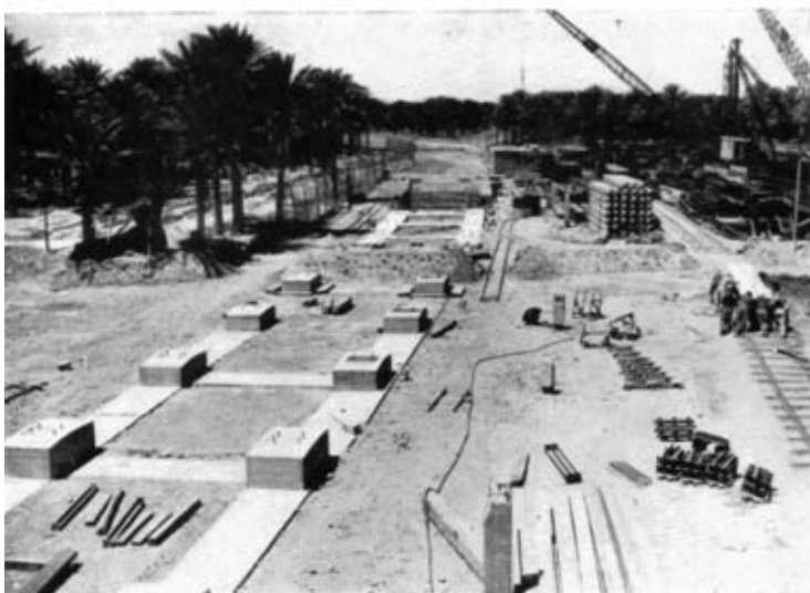
Photo 5. —Reinforced concrete rafts for approach viaduct foundations.
