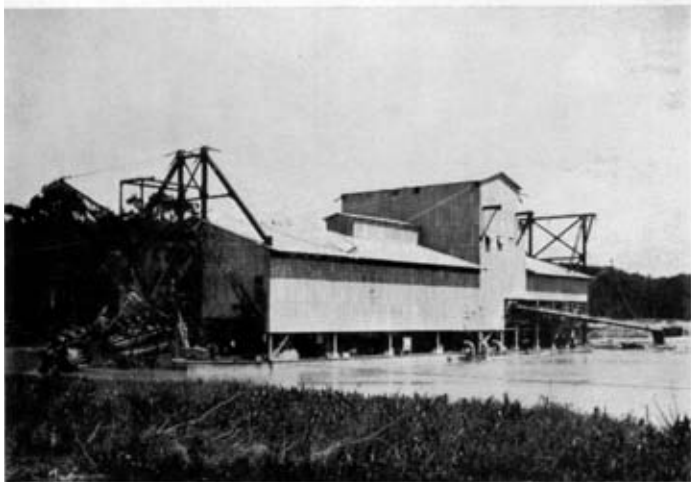
No. 4.—A tin dredge at work in central Malaya. Weighing over 800 tons, it floats in the pond which it creates by dredging virgin soil for extraction of tin.
