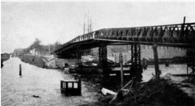
Photo 2. —“Iris” bridge at Stampersgat built by 756 Field Company. Originally constructed as 120 ft. double-single and 70 ft. single-single. The support on a skewed pier involved some cunning crib work. Photo shows the bridge after being raised by 1 Corps Troops to make the canal navigable for barge traffic.
