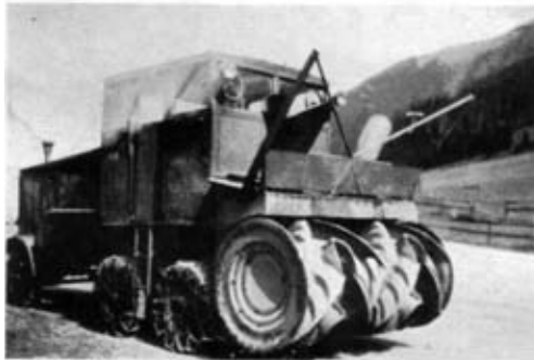
Photo 5. —Wheeled Schneefräse made by Laffley.
