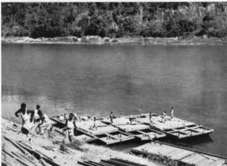
Photo 2. —Eastern Army boats under test load at Kalewa.
