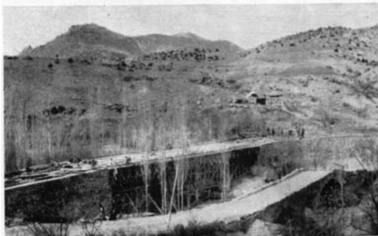
Photo 4. —Replacement of an old stone arch bridge by a Class 70 R.C. structure on road in Taurus mountains.
