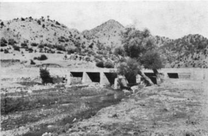
Photo 2.—Class 70 R.C. bridge replacing wooden bridge.
