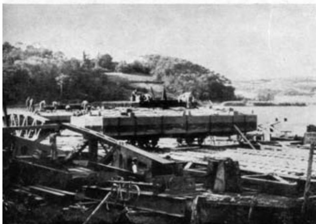
FIG. 44.—Erecting the girders on pontoons on a slipway.
