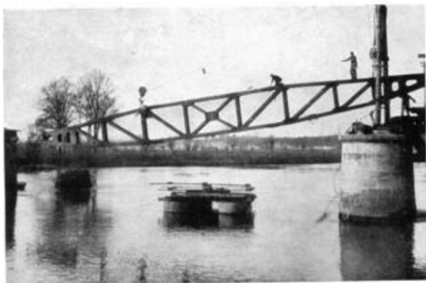
FIG. 39.—" Mulberry " component lengthened by the insertion of a central cross-braced panel.
