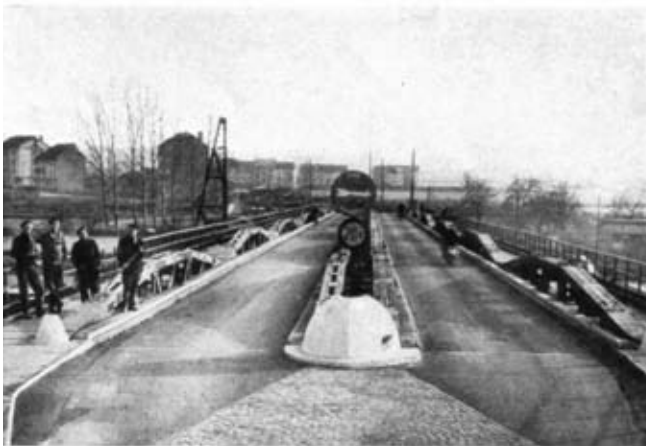
FIG. 32.—A "Mulberry" component bridge showing footpaths and hand-rails.
