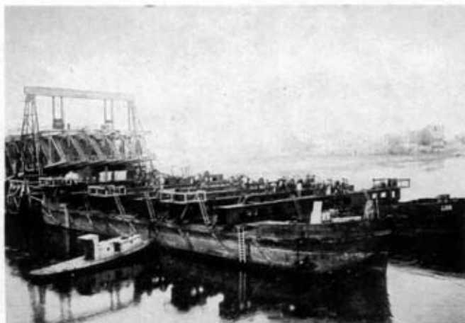
FIG. 4.—The first displacement of the suspension truss in preparation for its raising. The linked-up barges are grounded against the truss.
