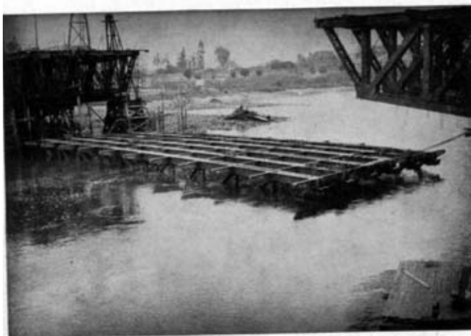
FIG. 6.—The truss at low water after its second displacement.
