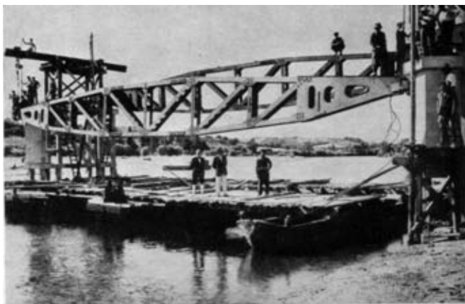
FIG. 37.—“ Mulberry ” spans carried on concrete trestles.
