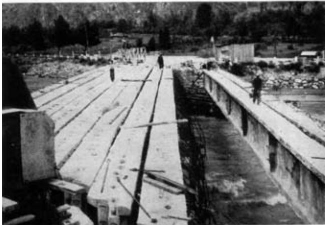
FIG. 20.—The final placing of the beams. The two beams on the right have still to be shifted. Note the cables for transversal prestressing passing through the top flanges.
