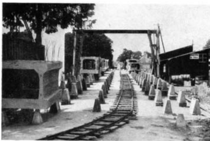
FIG. 26.—Finished voussoirs and arrangements for storage and transport
