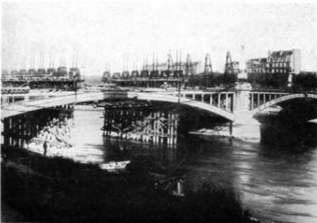
FIG. 16.—Arches back in final position.
