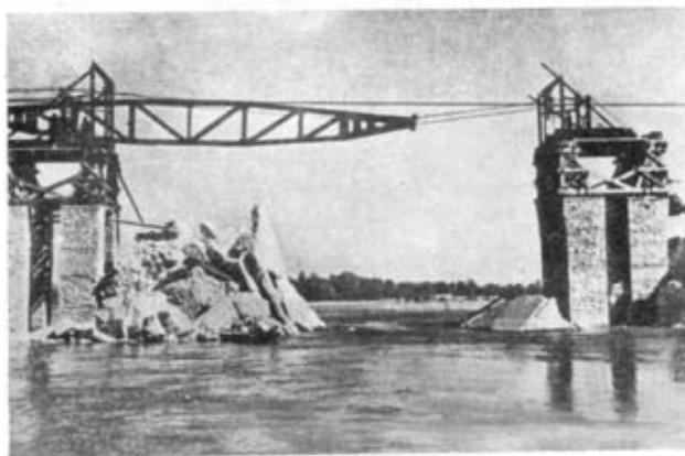
FIG. 40.—Cables guiding the front of the girder, which rested on a trolley at the rear.
