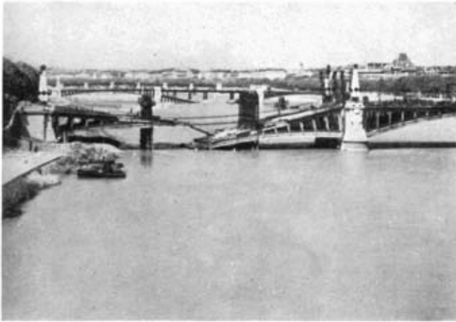
FIG. 15.—Lifting arches to final position.
