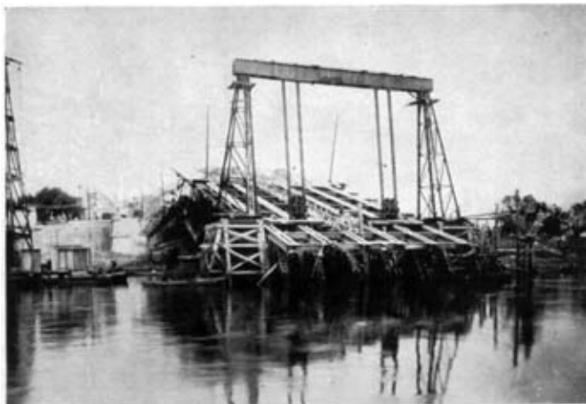
FIG. 3.—The general arrangement of the equipment used for raising the north cantilever.
