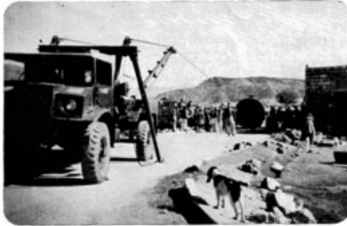
Photo 4.—Wana—1,500 gallon petrol tank being winched on rollers.
