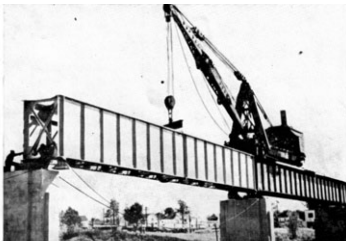
Photo 5.—Aluminium Alloy Railway Bridge Girder.
