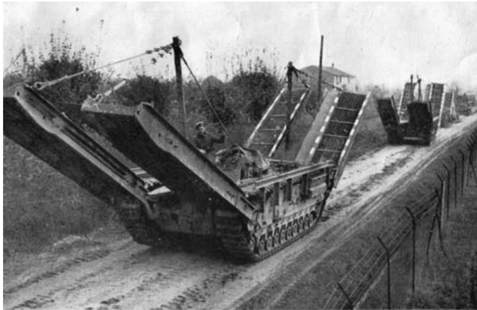
Photo 1. —ARKS moving along a road in Italy, showing metal treadway ramps, supported by king-posts.
