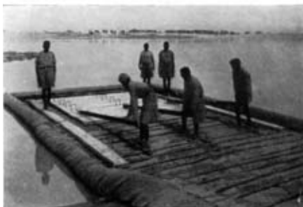
Photo 3. —Construction of the Indian Mat Bridge.
