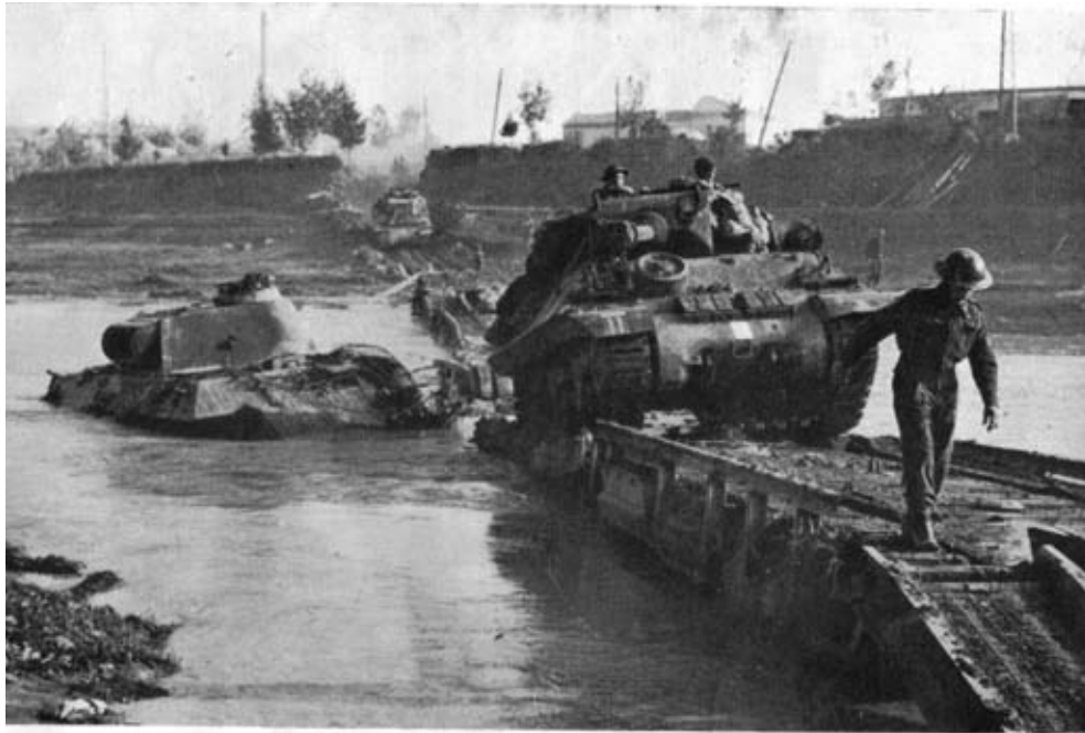
Photo 2. —Crossing the Savio at Cesena on ARKS. Width of water-gap, 200 ft. Depth in centre 5 ft.
