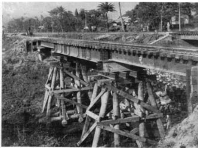
Photo 3. —Temporary piled bridge for new double line at Gauhati.
