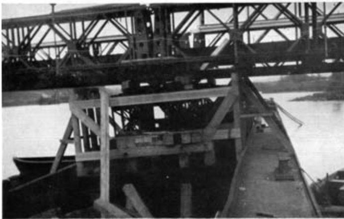
Photo 8. —Bristol Bridge. Wooden stability framework on the small barges.
