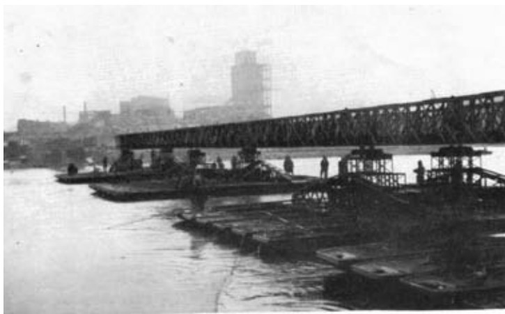
Photo 5. —Fulmar Bridge—booming out.
