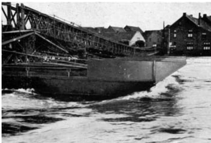
Photo 1. —Floods at Kent Bridge. Pier for double landing bay in 5\frac{1}{2} -knot current.
