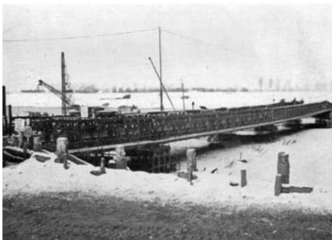
Photo 2. —Quebec Bridge, River Maas, Ravenstein. The southern approach spans showing the crib piers built on Chespaie-Sommerfeld bases. The latter bases are under the snow.
