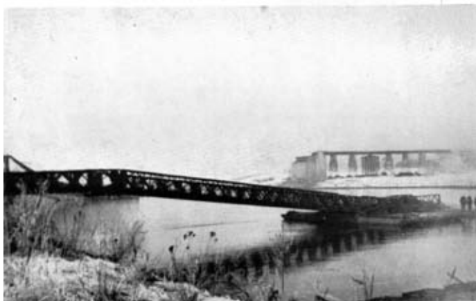
Photo 4. —Ilex Bridge. Launching a double landing bay. Six-pier raft just showing in right foreground, ready to be floated in.
