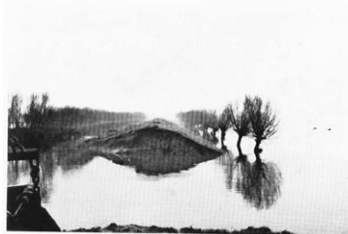
Photo. 4. —Breach in main flood-bank at Crowland causing flooding of 35,000 acres of agricultural land (shown on right).
