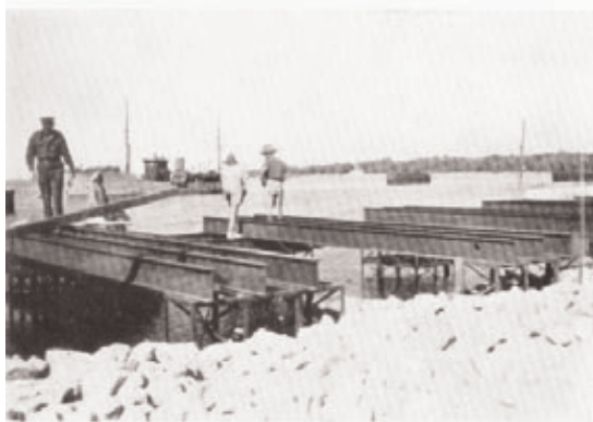
Photo 5.—Temporary lighter wharf.
