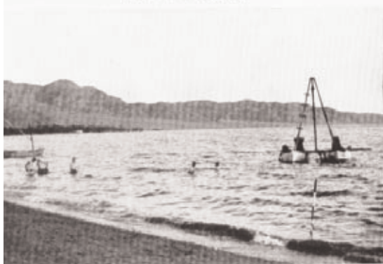
Photo 2.—AKABA. Boring rig on boats.
