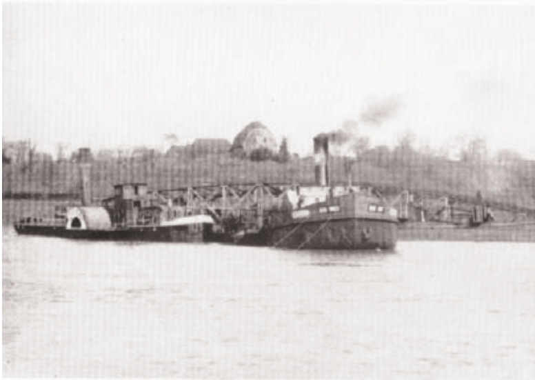
Fig. 3. —Usen Bridge raised on barges with tugs Oker and Widder.
