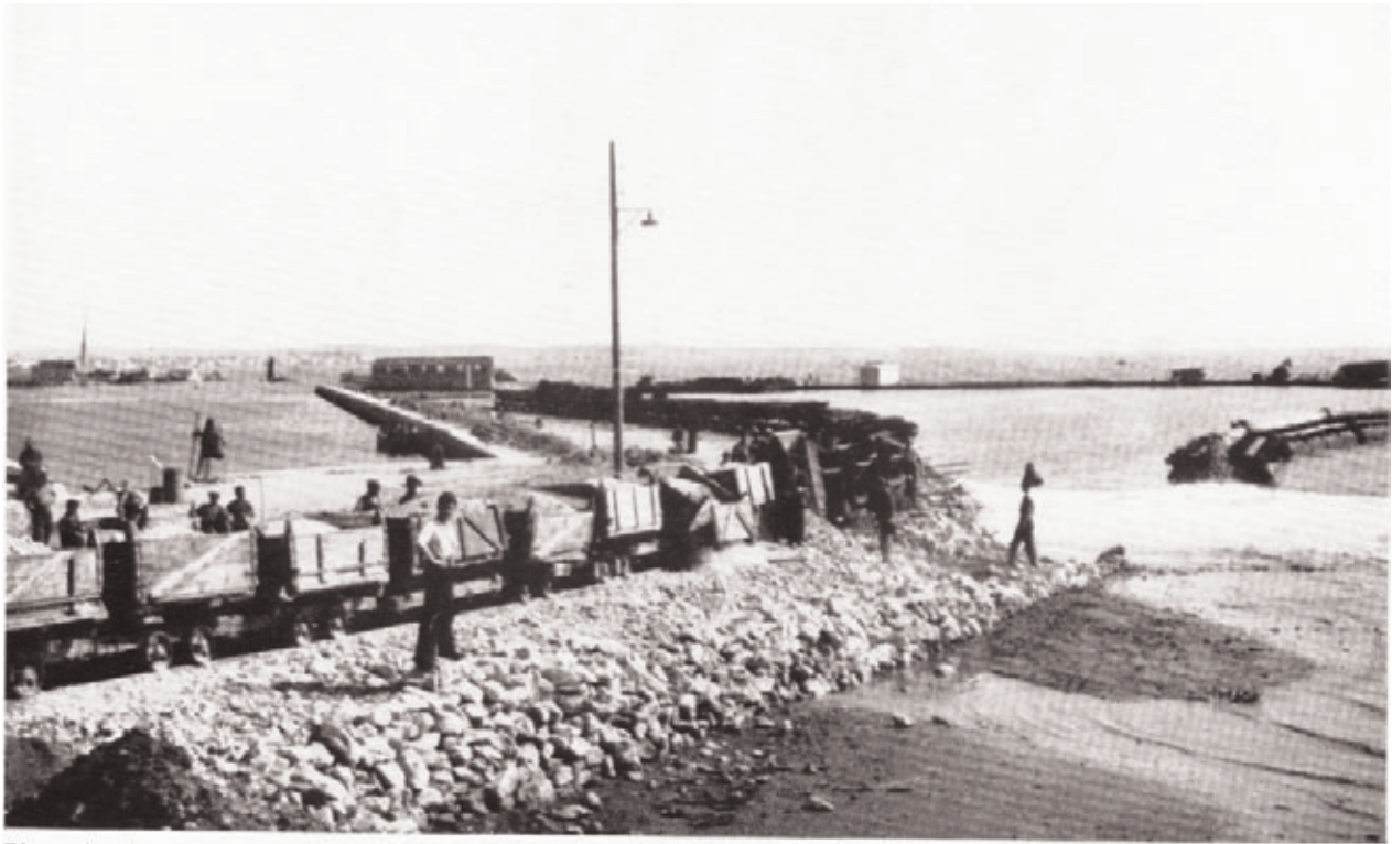
Photo 4.—A general view of the new quay during construction. The 24" delivery pipe line from the dredger Strymon can be seen on the right.
