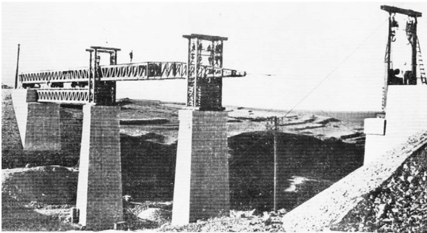
Photo. 4.—Haifa-Bairut-Tripoli Railway. Launching Unit Construction Railway Bridge spans.
