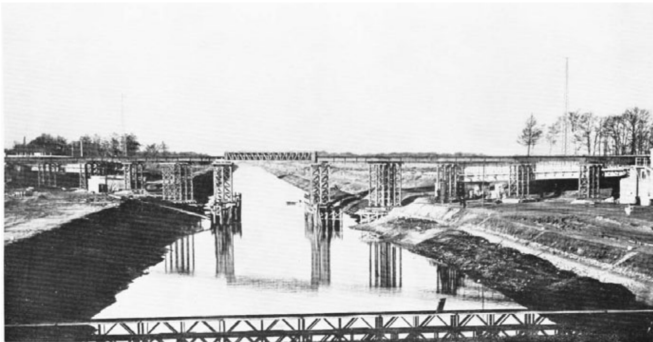
Photo. 3. —Bridge over the Albert Canal at Herenthals. View after reconstruction, with U.C.P.B. Through Span, 40 ft. Sectional Bridge and Standard Trestling.
