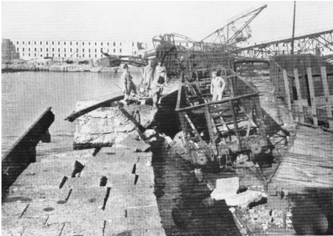
Photo. 1. —Naples after occupation in September, 1943. Repairs to damaged Quay face, in progress.
