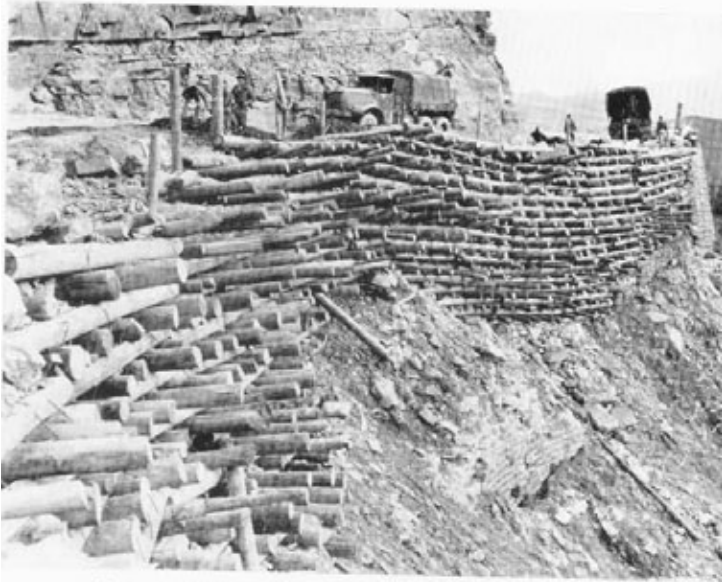
Plate 7.—Timber cribbing on Route 67 in Northern Apennines.
