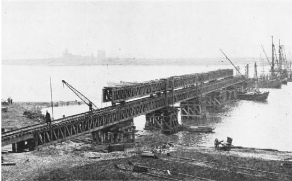
Railway bridge over the Rhine at Spyck. Spans in position and ready for launching.
