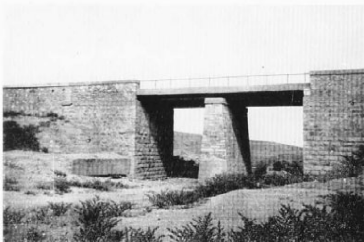
Plate 8.—ASVESTOKHORION BRIDGE Abutments rebuilt from foundations upwards. Centre pier added and gap spanned by R.S.J.s and concrete.
