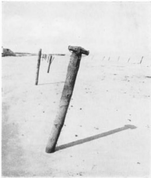
Pile with Teller Mine Attached to Top. (Picture taken at low tide.)
