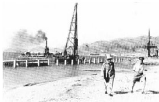
Photo 3.—Driving Reinforced Concrete Piles. Personnel Camps in Background.
