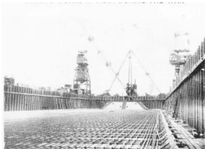
Reinforced concrete floating dock at Cocanada. Reinforcement for bottom in position preparatory to pouring.
