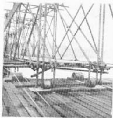
Fig 11.—Wheeled bearing of the bridge.
