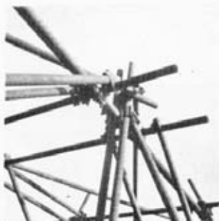
Fig 3.—Top chord's joint.
