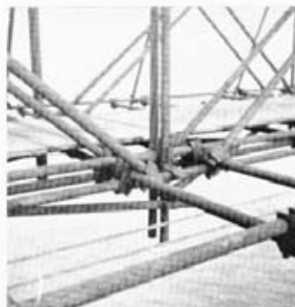
Fig 6.—Bottom chord's joint.
