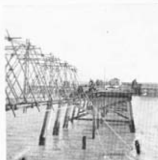
Fig 4.—The bridge in launching (ropes just being dismantled).
