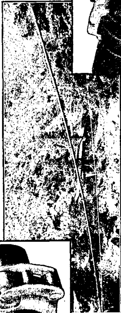
Air main with Victaulic Joints slung on two steel cables across the gorge of the Hikone River, Japan. View shows a 200-ft span of 8-in. line.
