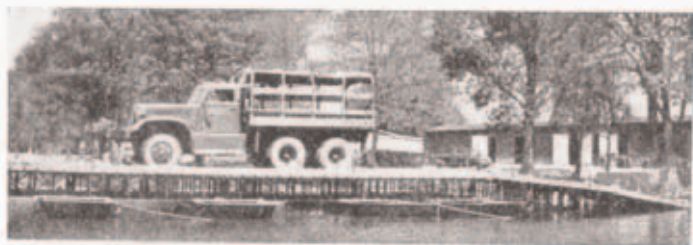
Pontoon Bridge Constructed of Half-Boats and Light Trusses.
